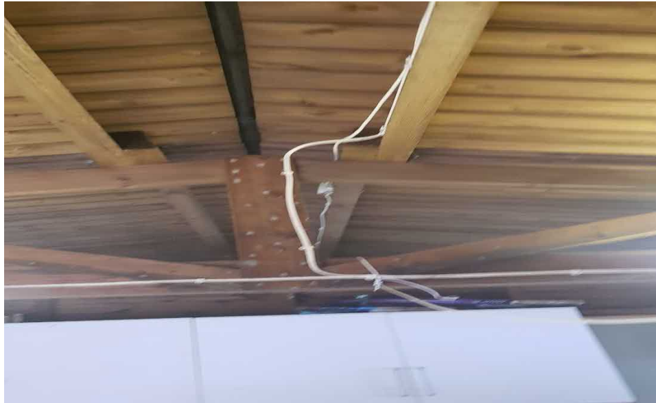
Picture 3: Showing the internal structure of the double garage
