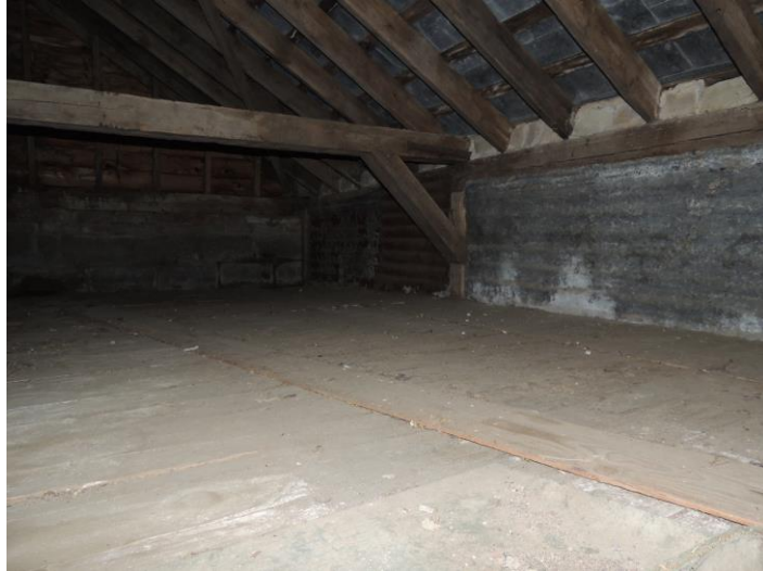
Photo 10: Note lack of evidence of bats on mezzanine floor
