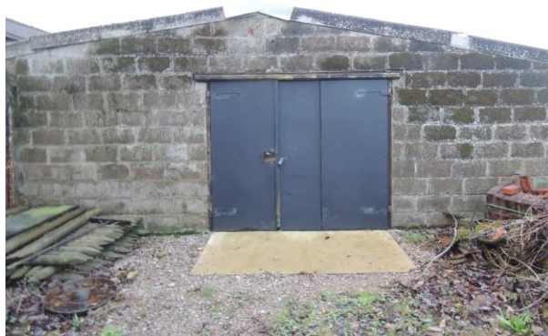
Photo 2: North-eastern end of former farrowing shed
