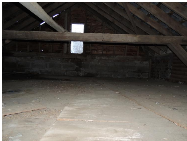
Photo 9: Note lack of evidence of bats on mezzanine floor
