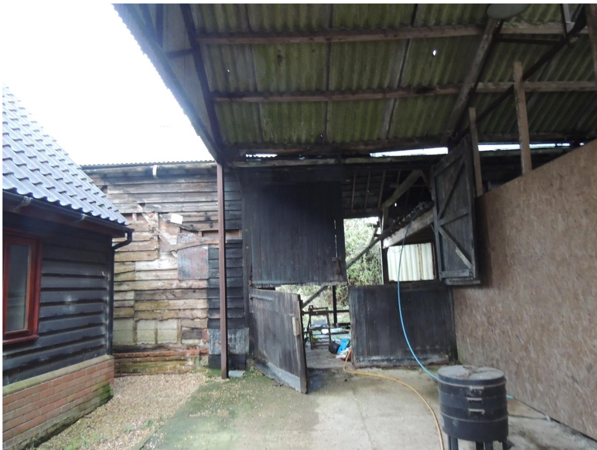
Photo 1: Looking towards the eastern elevation of the barn
