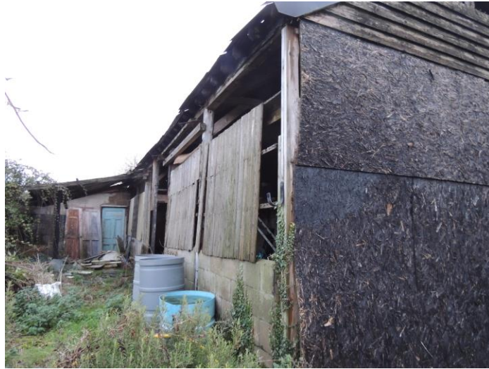
Photo 4: South-western end elevation of barn, north-western side (note gaps in walls) and, at far end, south-western end of farrowing shed
