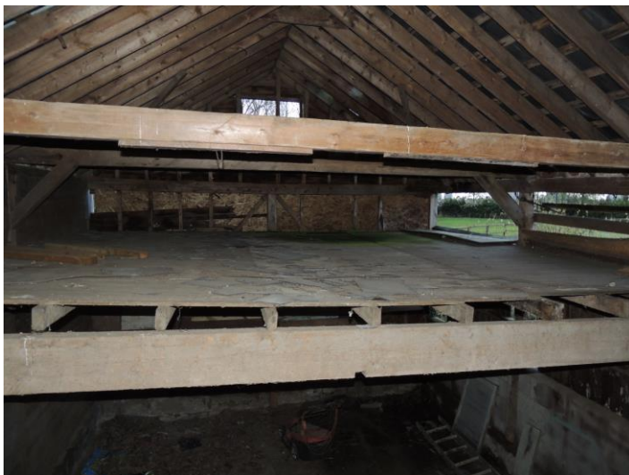
Photo 12: Note lack of evidence of bats on mezzanine floor
