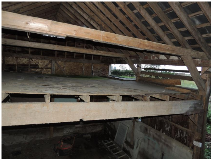
Photo 13: Note lack of evidence of bats on mezzanine floor
