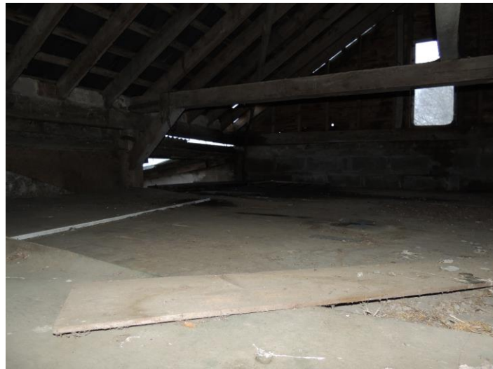
Photo 11: Note lack of evidence of bats on mezzanine floor
