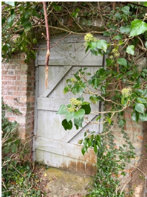
The existing opening and gate in the east wall of the lower garden. The opening is older, the joinery is modern
