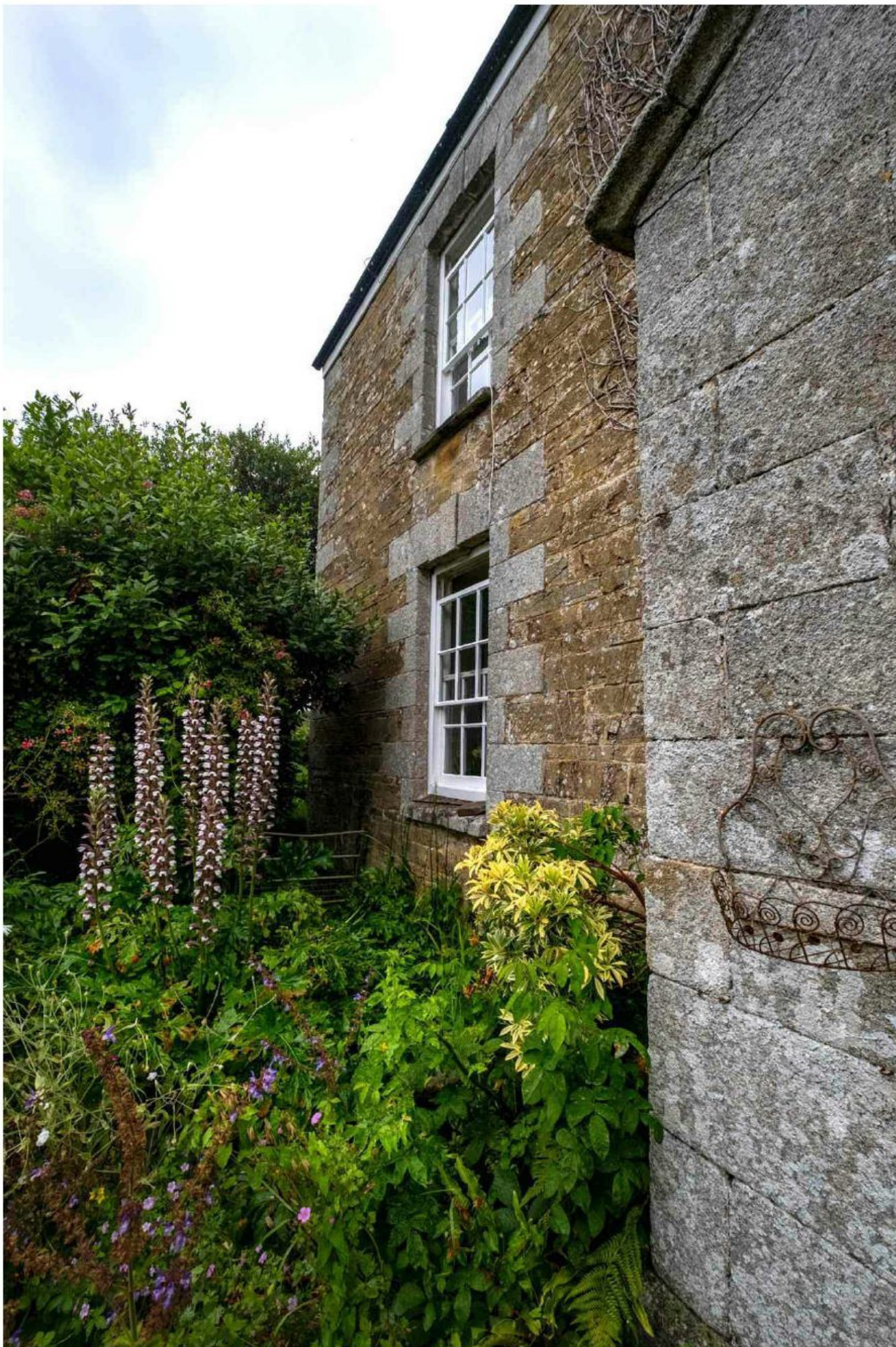
Detail showing the stone on the 'show', south elevation. The cavetto moulded copings to the granite ashlar porch are seen
