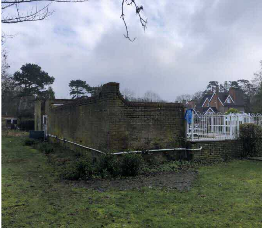
Existing Perimeter wall to Swimming Pool area
