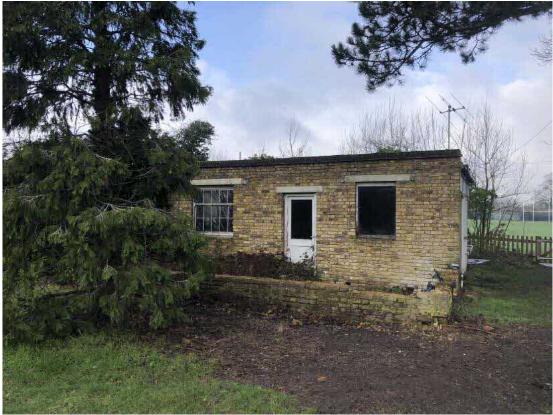
Existing Outbuilding number 2 for removal
