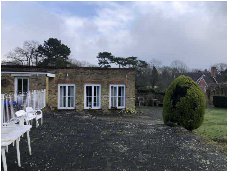
Existing Paving with main house behind
