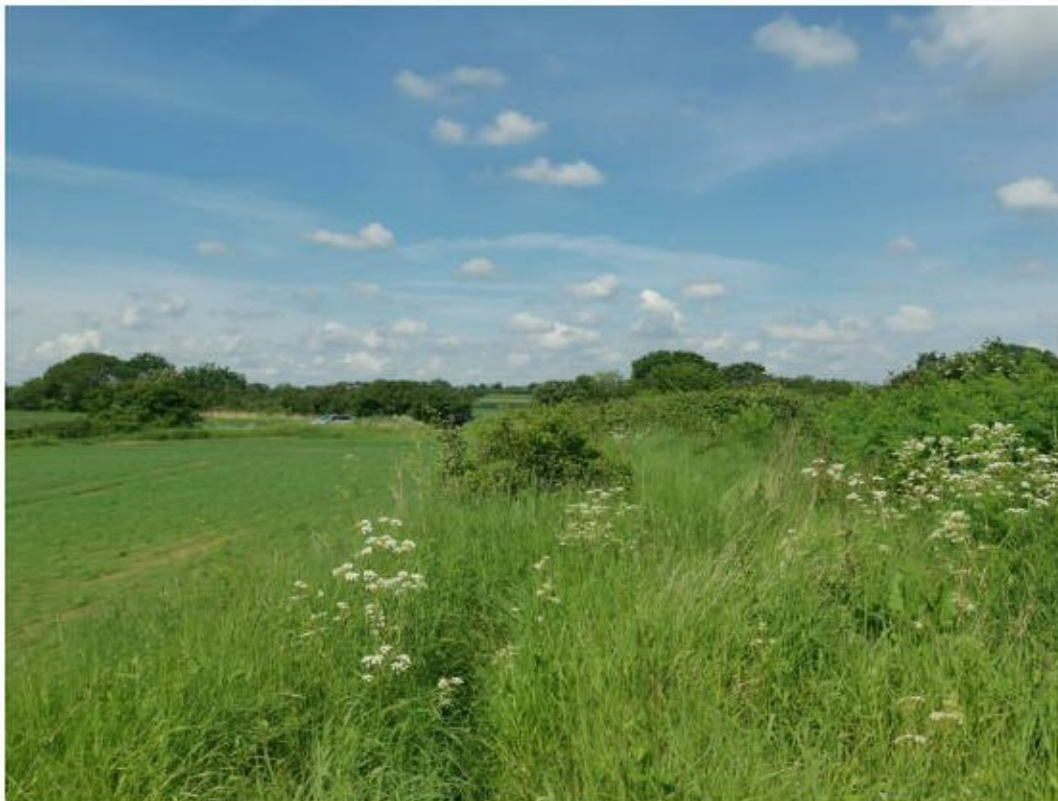
Photograph 2 – View of central grass bund, facing west.
