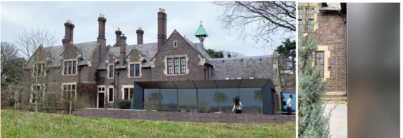
Figure 4: Glazed rear extension elevation and photographs from southeast and cladding sheen finish
