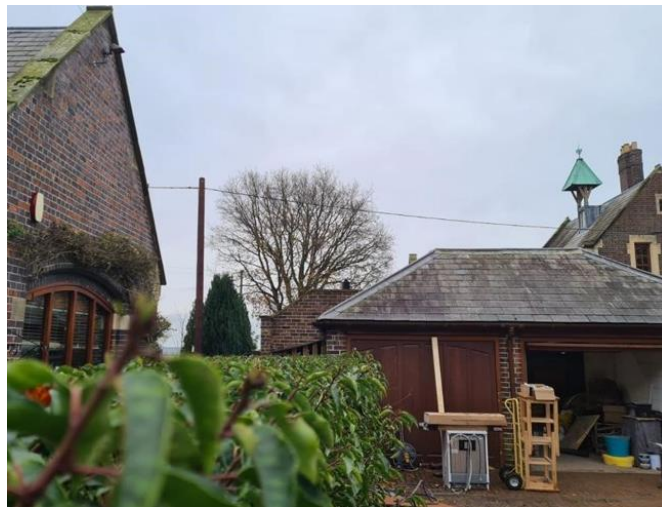
Figure 10: View of parapet wall from front elevation
