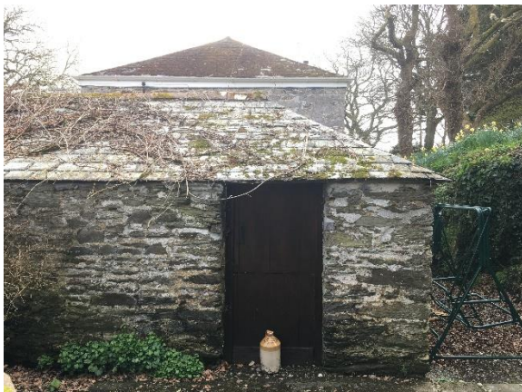
Northern end of Out-Building / Store [proposed Dining space]
