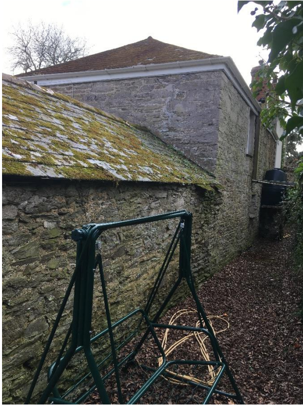
Western flank wall of Out-Building range and House
