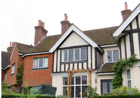
Detail of south elevation roof
