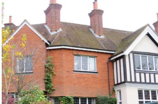
Detail of south elevation roof
