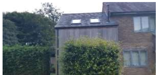
South East end of the front of the house
