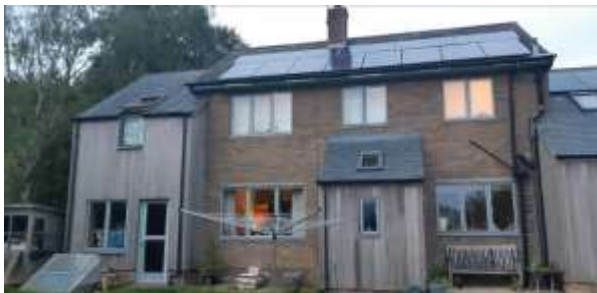
Rear of the house
