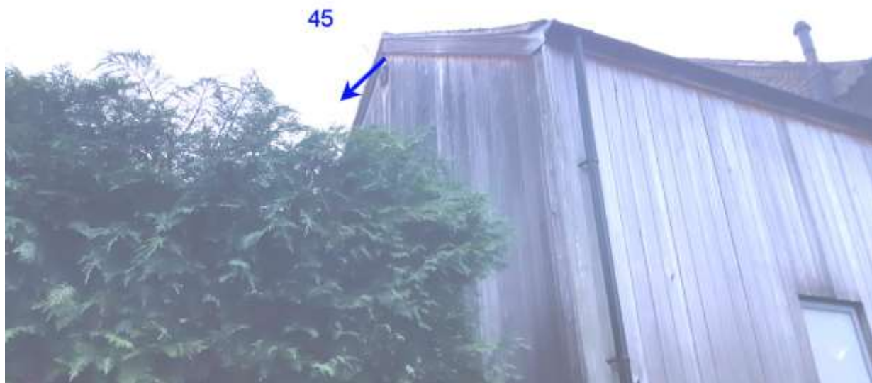
Common pipistrelle roost on southern end of the building.
