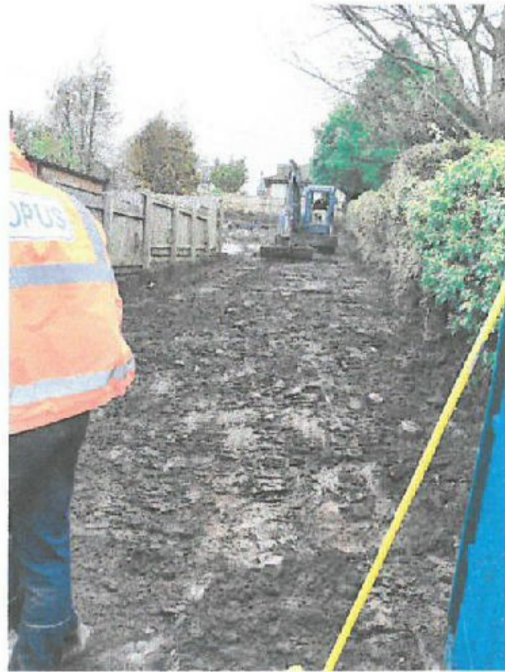
Photo 2 depth of excavations proximal to T1- T3 taken by Mrs Henderson 27.10.21
