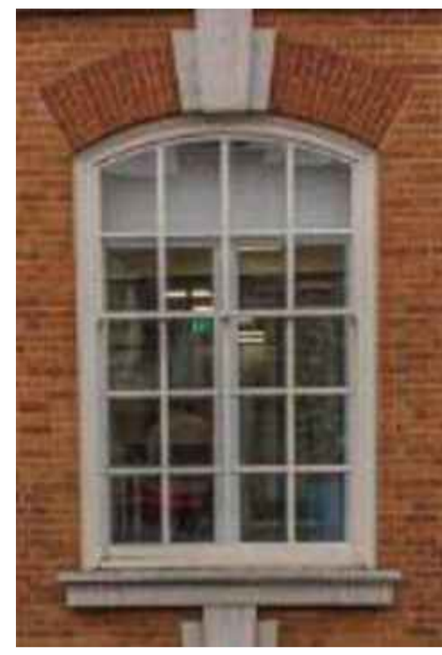
2 PHOTO FROM STEEL WINDOW NTS
