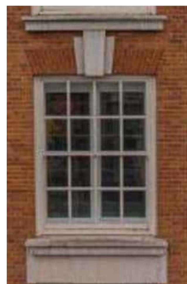
2 PHOTO FROM STEEL WINDOW NTS
