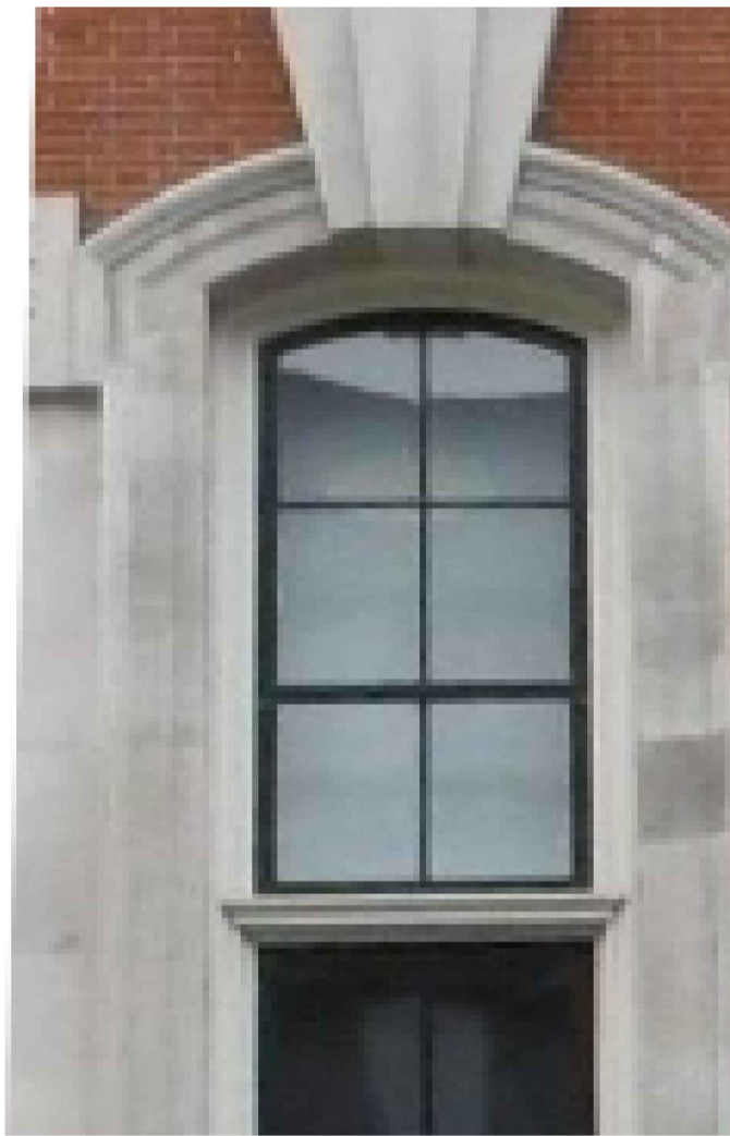
2 PHOTO FROM STEEL WINDOW NTS
