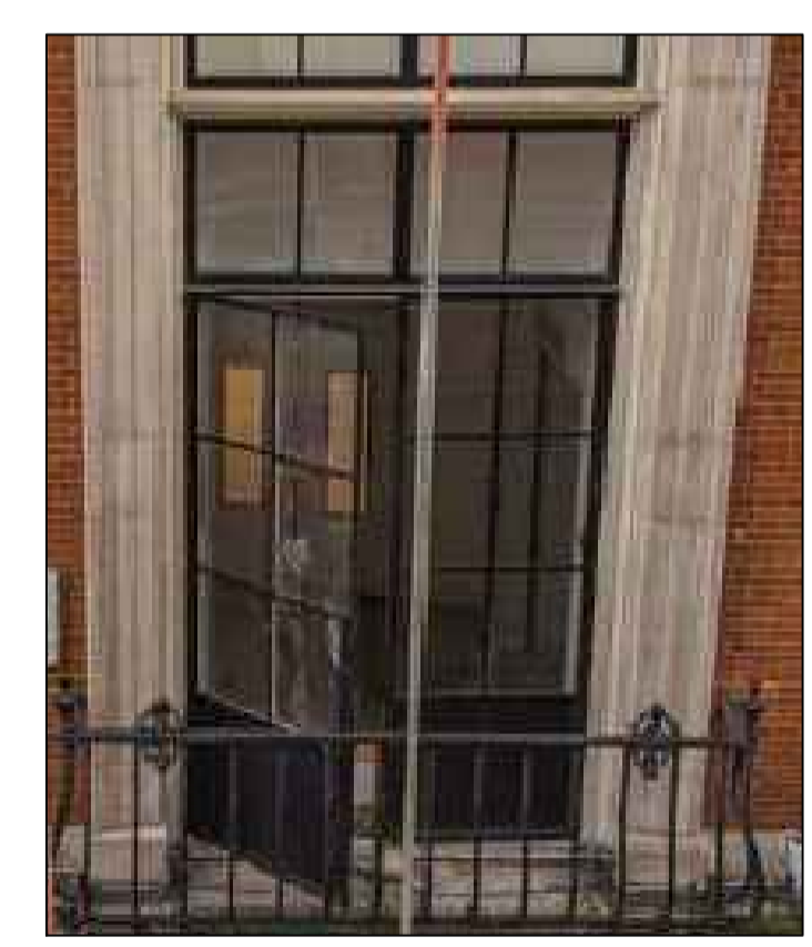
2 PHOTO FROM STEEL WINDOW NTS
