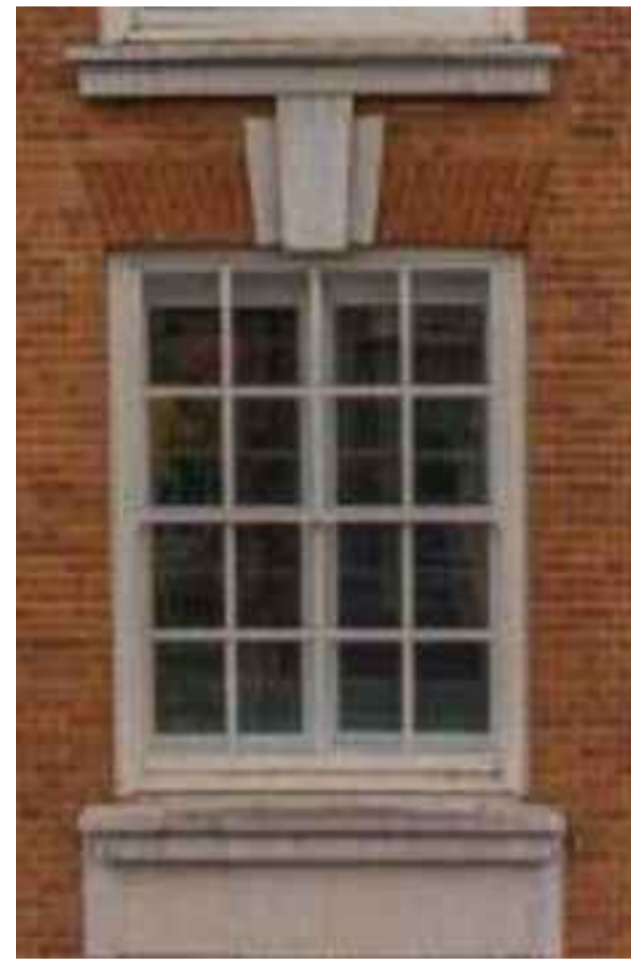
2 PHOTO FROM STEEL WINDOW NTS
