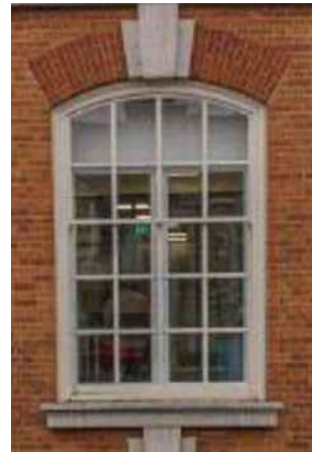
2 PHOTO FROM STEEL WINDOW NTS
