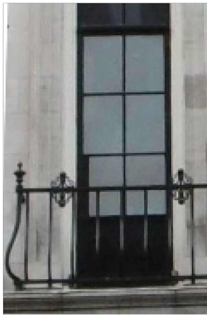
2 PHOTO FROM STEEL WINDOW NTS
