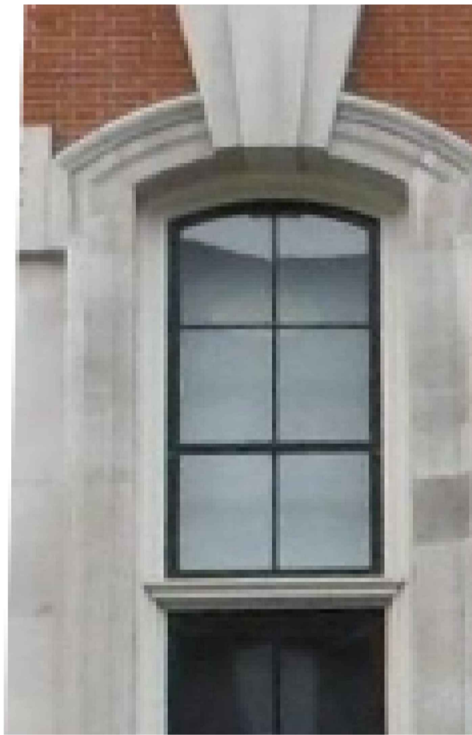
2 PHOTO FROM STEEL WINDOW NTS
