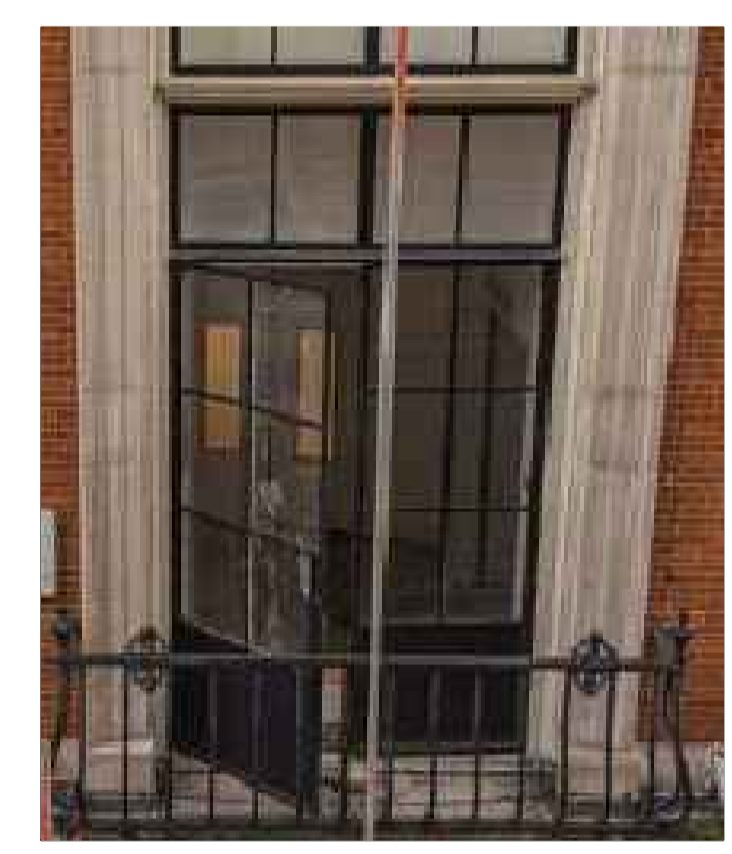
2 PHOTO FROM STEEL WINDOW NTS
