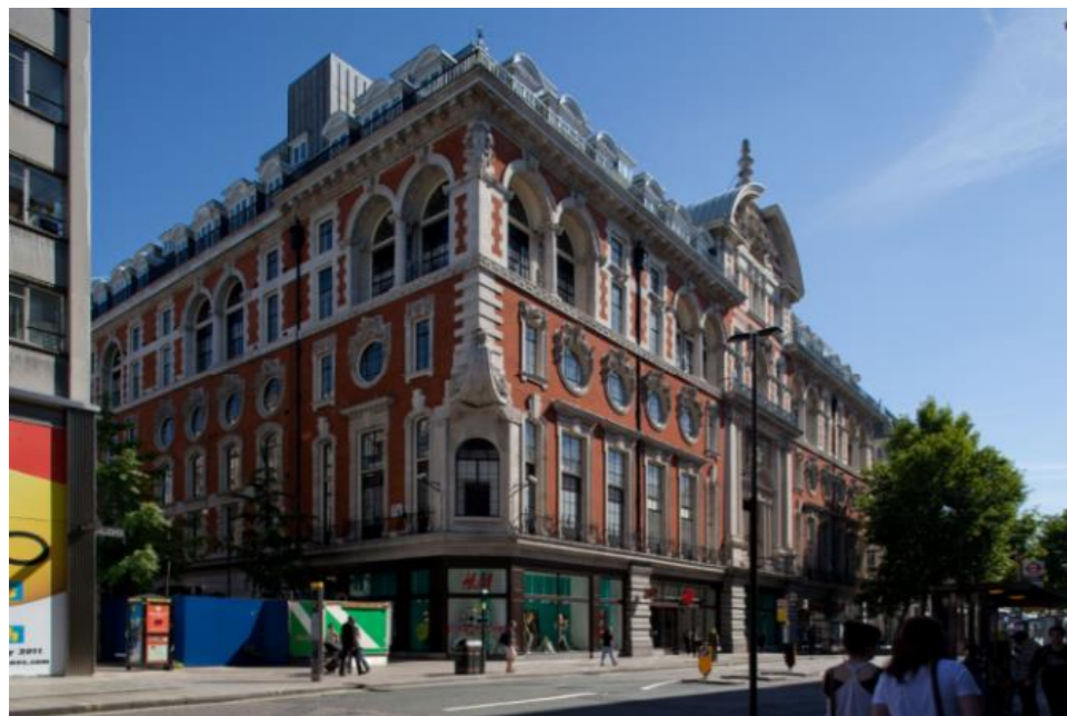
Above: permitted modifications to UK House's mansard roof
