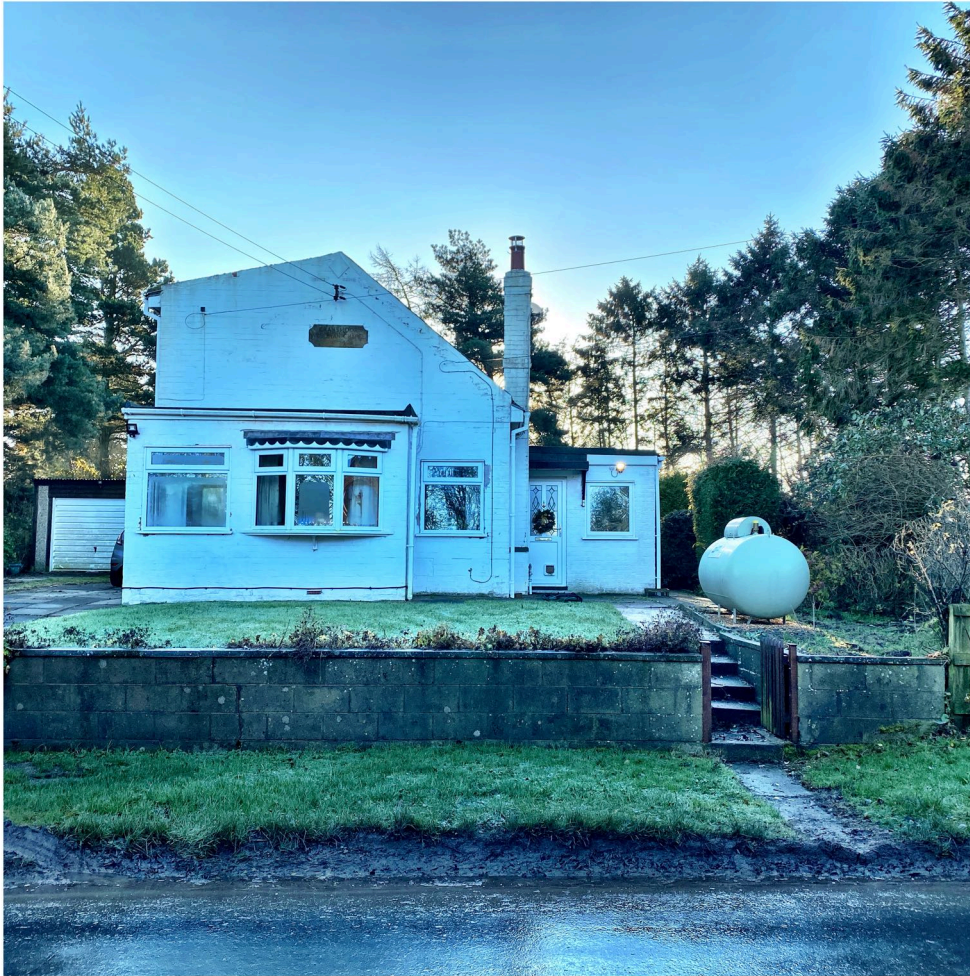
Close-up View of Installation
