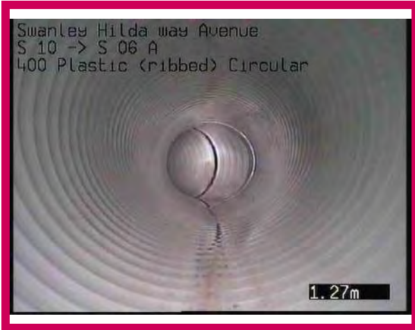
1, 00:00:08, 1.27 m General remark, Photograph: Pipe condition
