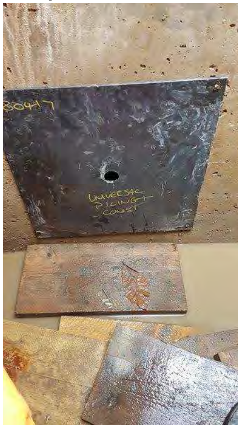
Fig D.2 – Orifice Plate Installation 2
