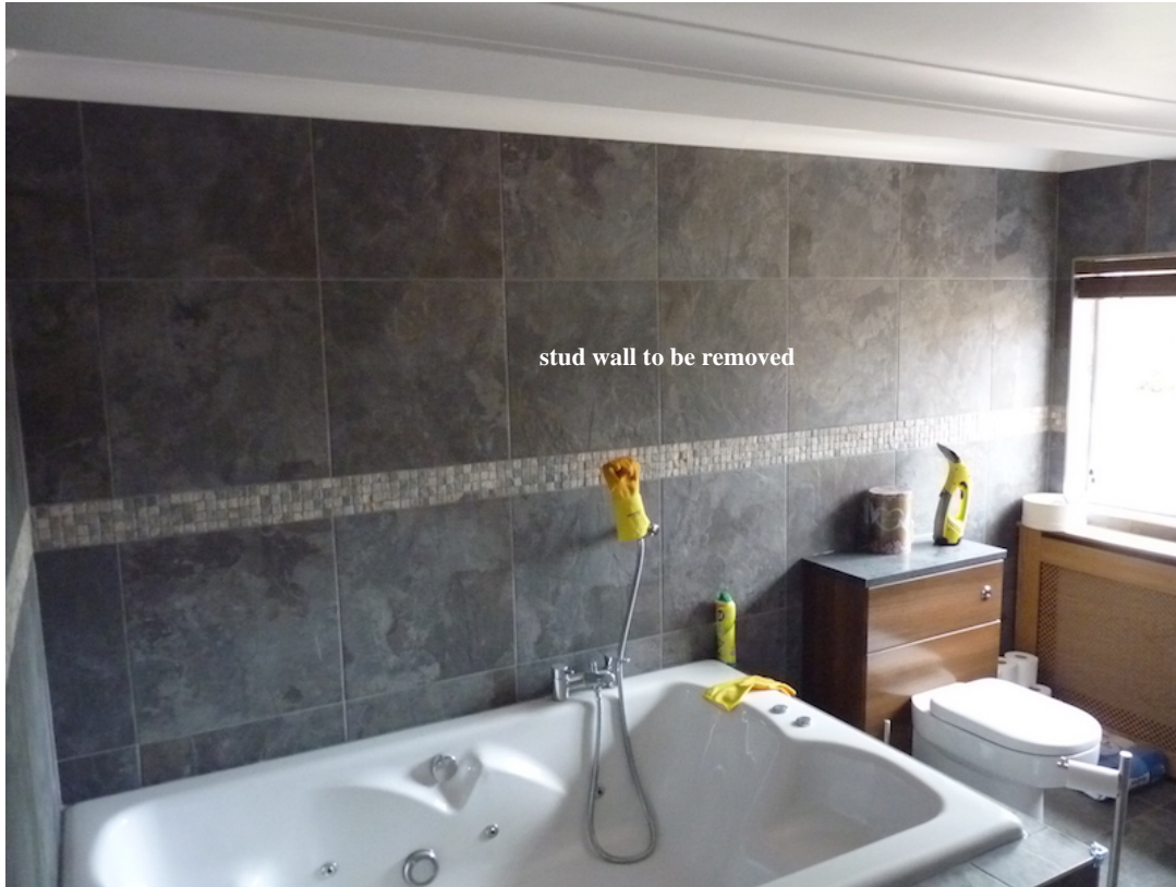
Photo within master bathroom facing stud wall to be removed
