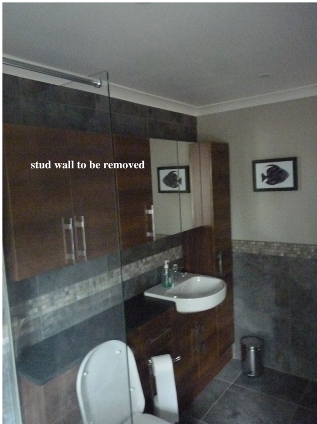
Photo within family bathroom facing stud wall to be removed
