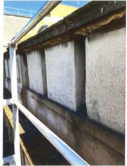
Fig 46: Precast balustrade sections
