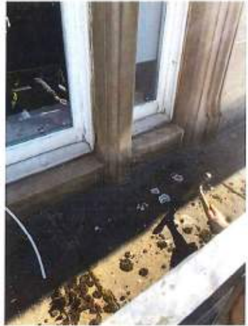
Fig 66: 4 th floor cill tap testing
