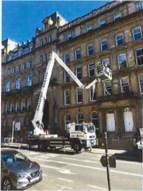
Fig 41: Survey in progress
