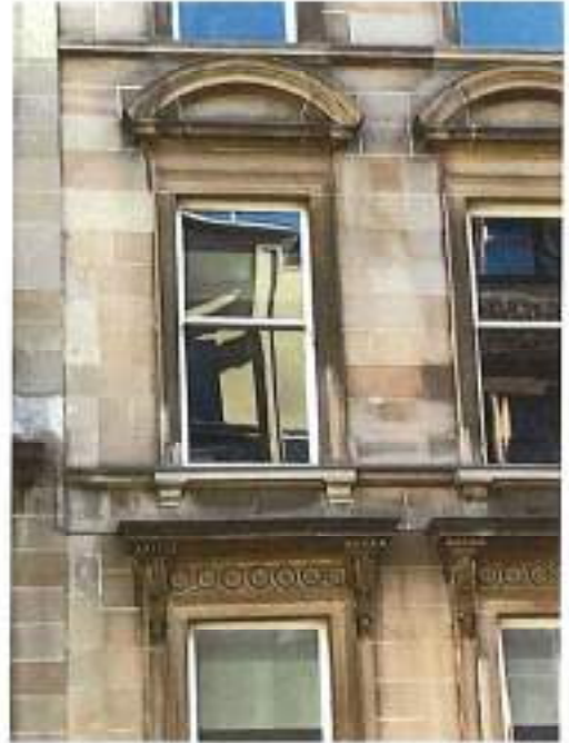
Fig 14: 2 nd floor level
