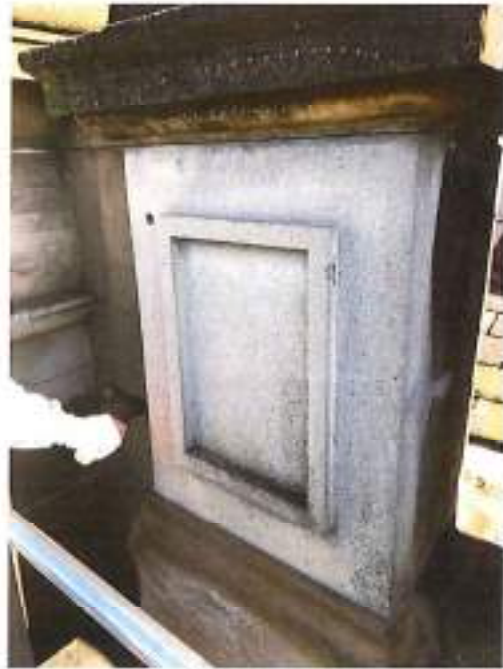
Fig 60: Part replacement with concrete
