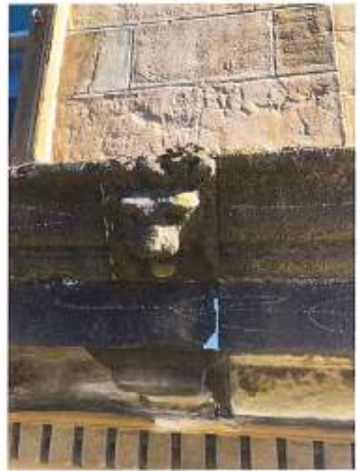
Fig 72: 4 th floor projecting cornice
