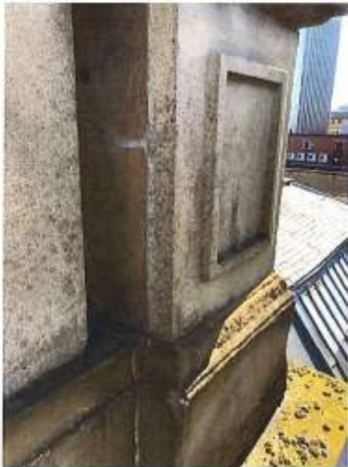
Fig 47: Part replacement with concrete
