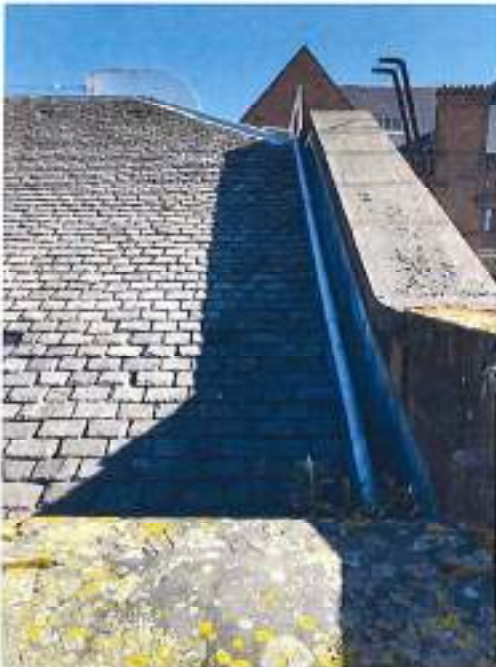
Fig 43: Overview of roof
