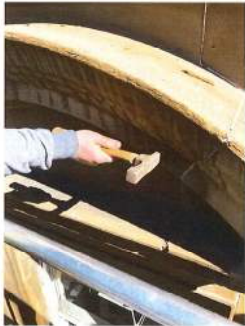
Fig 92: Tap testing 2 nd floor hoods
