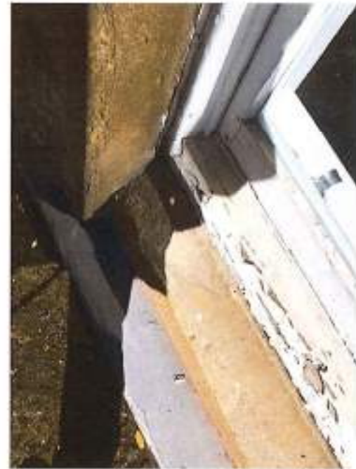
Fig 106: Corroded cramps parapet cope (Portico)
