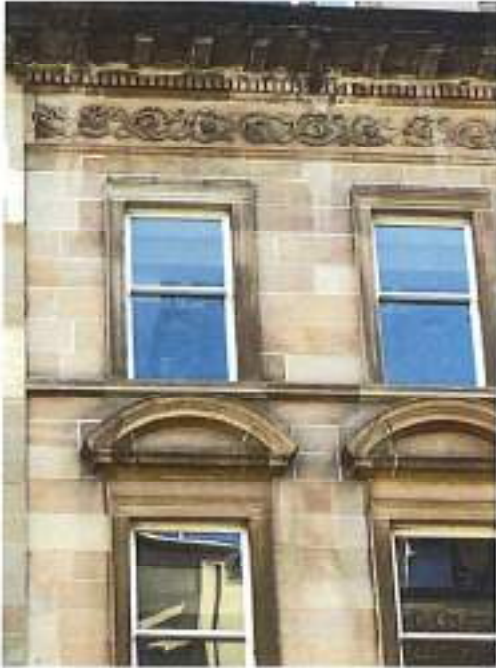
Fig 13: 2 nd Floor level
