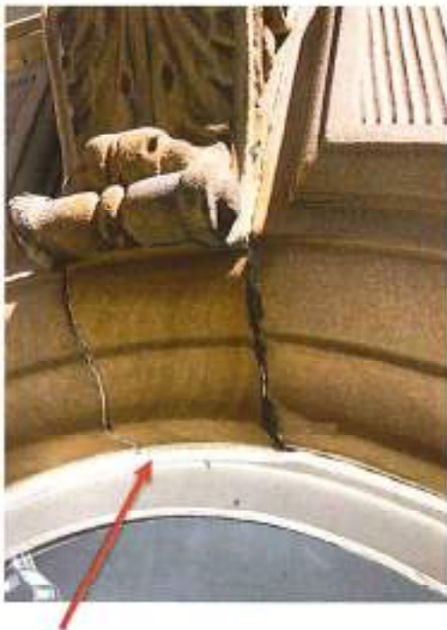
Fig 119: Movement to centre arch detail (Keystone)
