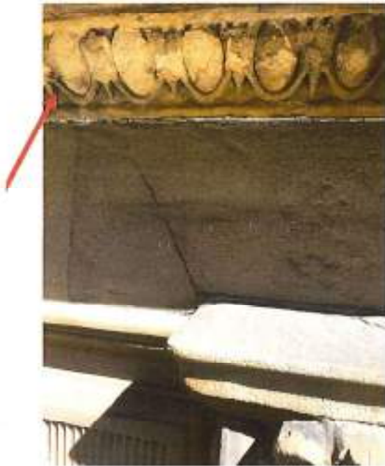
Fig 115: Egg & dart mould GL friable
