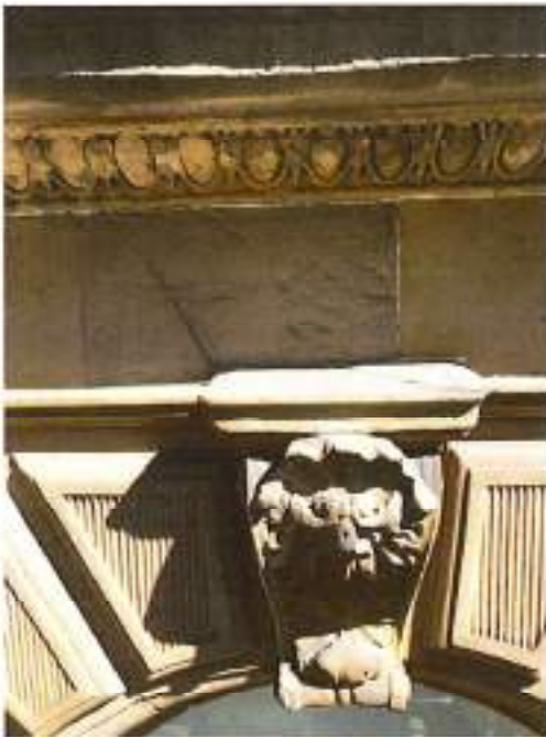
Fig 111: Ground floor window detail
