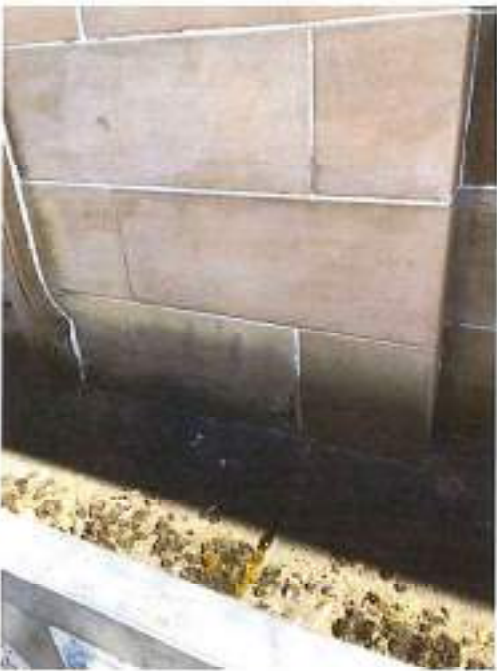
Fig 67: 4 th floor projecting cornice
