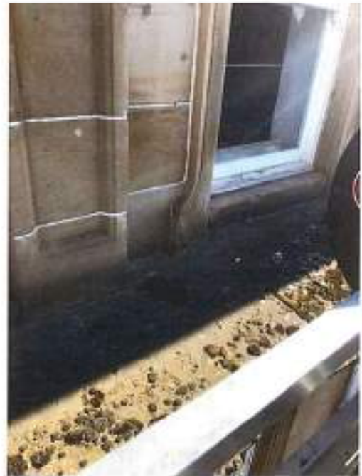
Fig 68: 4 th floor projecting cornice
