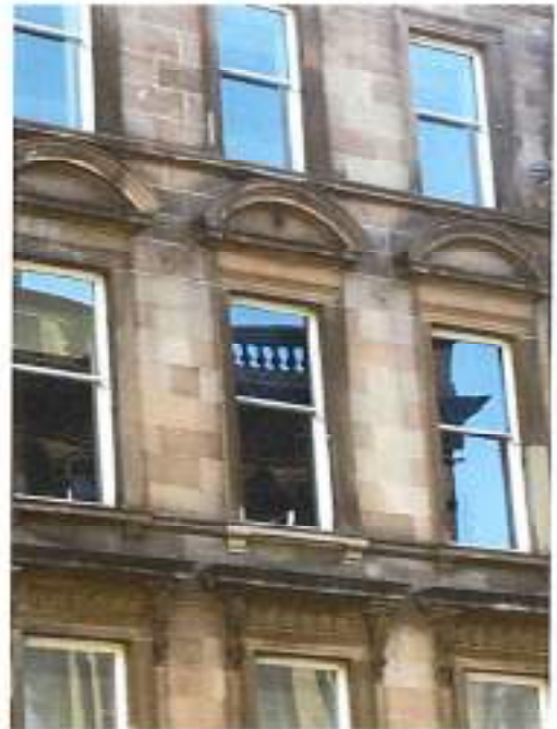
Fig 6: 2 nd Floor level
