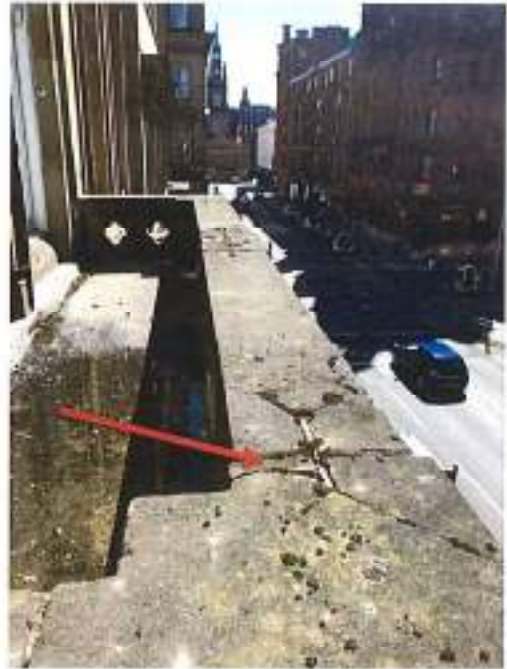
Fig 106: Corroded cramps parapet cope (Portico)
