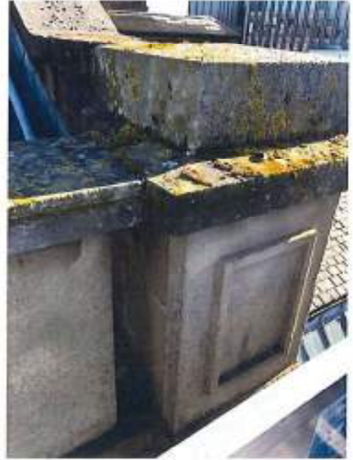
Fig 42: Parapet at roof level
