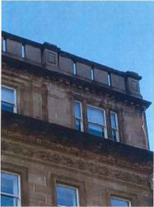
Fig 5: Balustrade course at roof level
