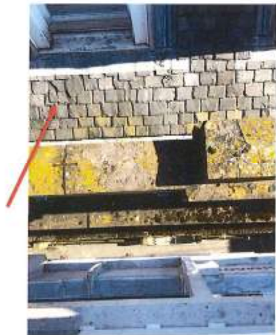
Fig 56: Slipped/moved slates
