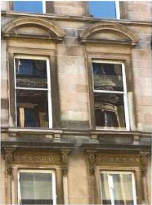
Fig 15: 2 nd Floor level
