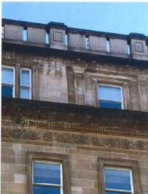
Fig 3: Balustrade course at roof level
