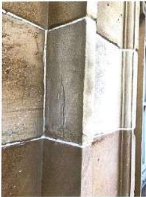
Fig 69: Small fissure
