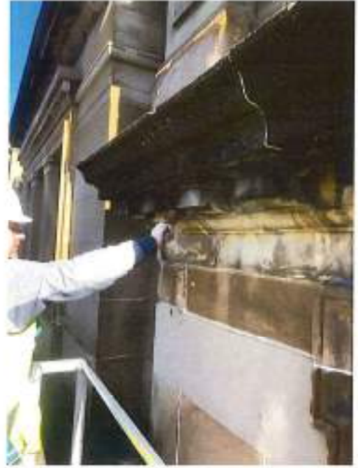
Fig 62: Tap test in progress Eaves projecting cornice
