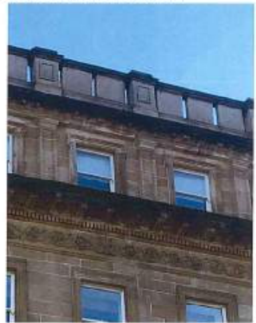
Fig 4: Balustrade course at roof level
