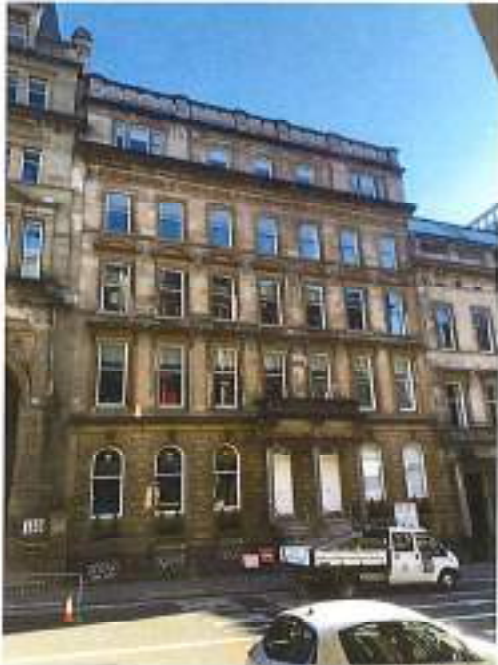
Fig 1: Front elevation from ground
