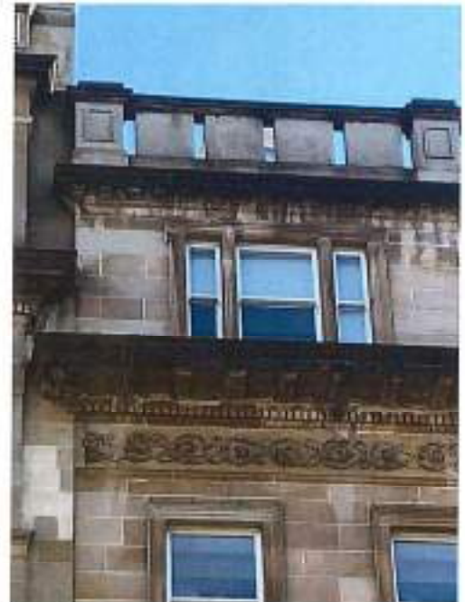
Fig 2 : Balustrade course at roof level
