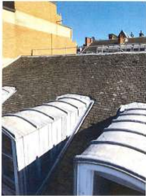
Fig 57: Overview of roof
