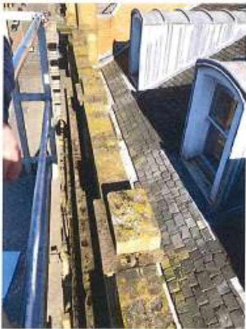
Fig 59: Overview of roof
