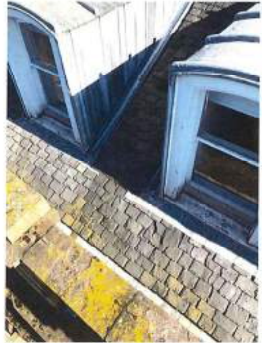
Fig 58: Overview of roof
