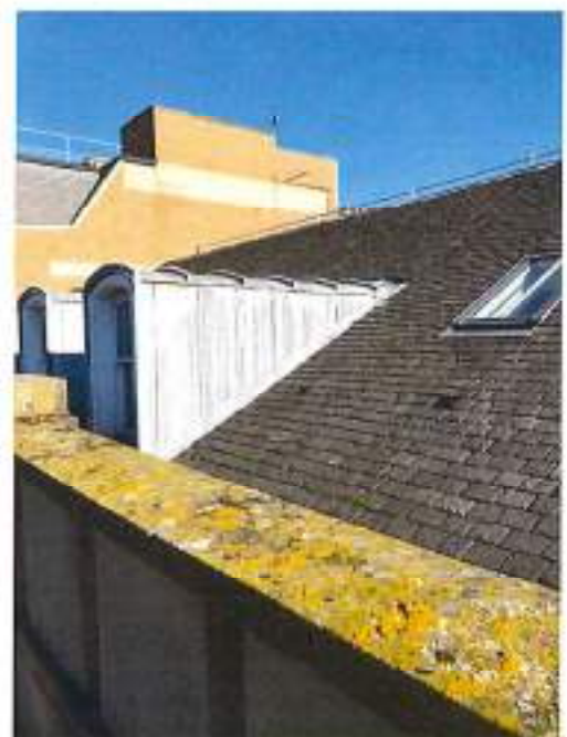
Fig 44: Overview of roof
