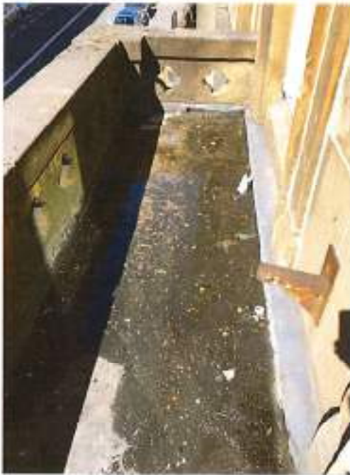
Fig 107: Portico roof behind parapet
