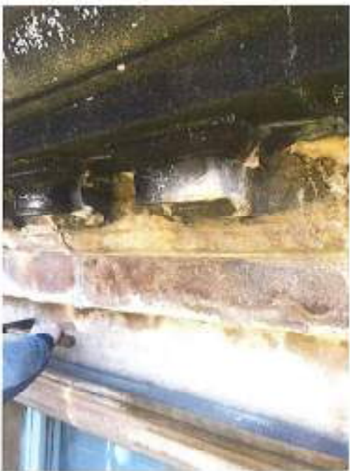
Fig 71: eaves level projecting cornice
