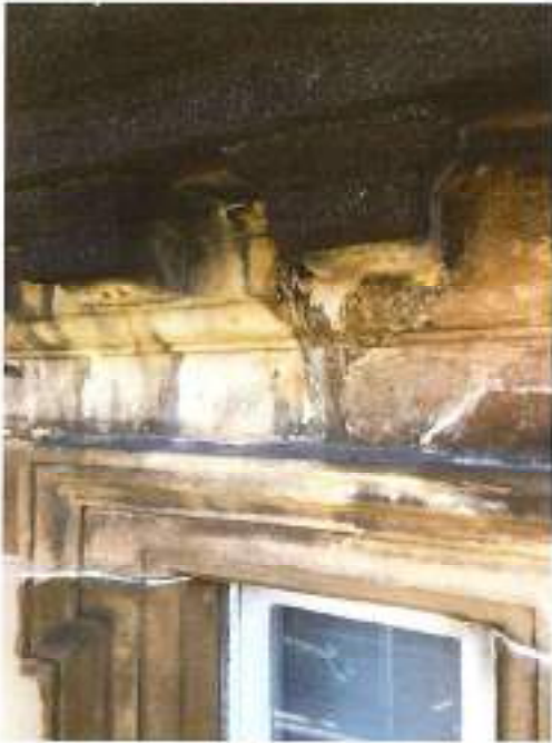
Fig 63: Underside eaves projecting cornice
