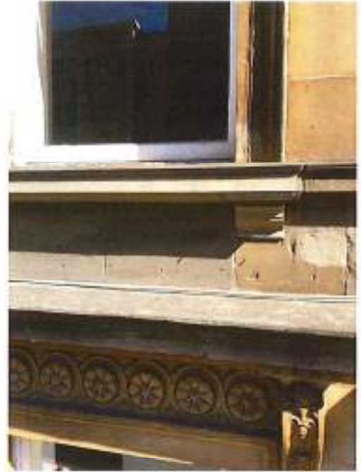
Fig 102: New cill 2 nd floor
