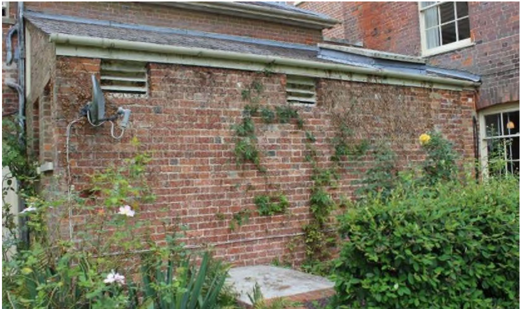
Figure 24 The lean-to housing the bread oven, south-west elevation.
