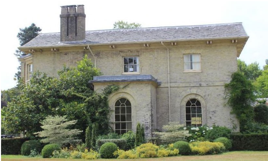
Figure 16 North-east elevation of the Nash house.
