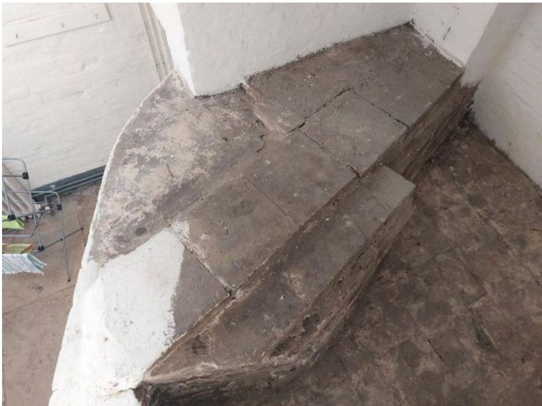
Figure 44 The flue from the oven chamber runs across the top of the oven to a chimney, now capped, on the north-west wall.
