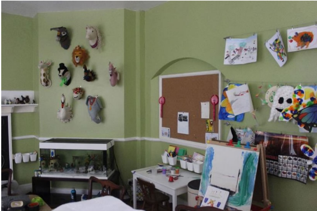
Figure 49 The blocked door that linked the 'occasional room' to the now demolished servant's hall.
