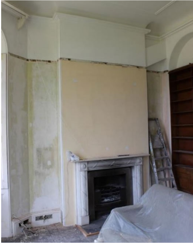
Figure 34 The room at the south-west end of the garden front.
