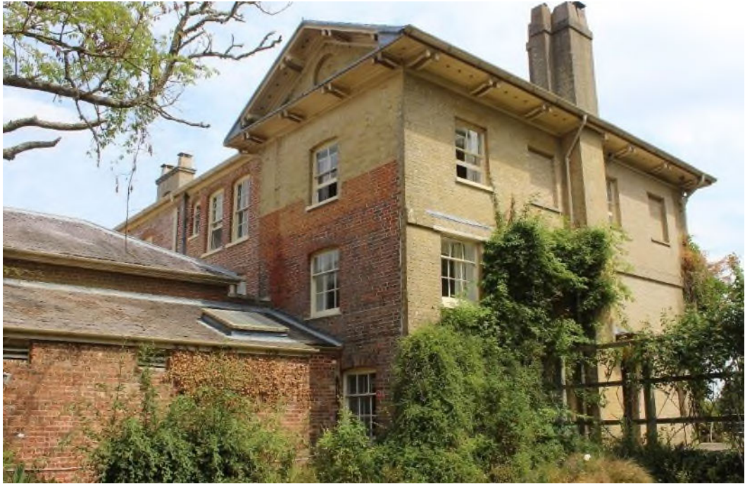
Figure 22 The north-west elevation of the south-western element of the house.
