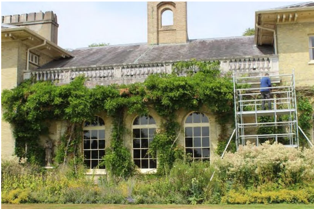
Figure 18 South-east elevation, central single storey element remodelled by P.S. Webb in 1898/9.
