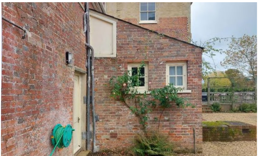
Figure 25 The north-west elevation of the bread oven building.
