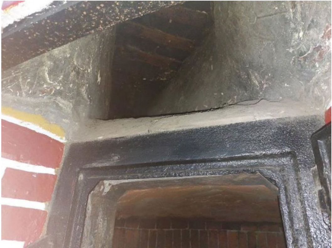
Figure 43 The flue opening above the oven door.
