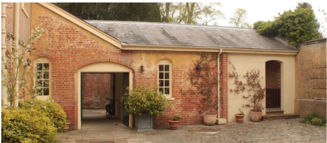
Figure 27 The remnant of Webb's service range, originally a bicycle store to the left of the arch and a space described as 'occasional room' to the right which was accessed through a blocked door now within the rendered section of wall.
