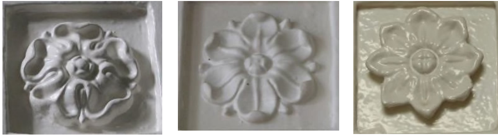
Figure 31 The flower heads used to decorate the top corners of the doorcases; left: main entrance hall/stair compartment; centre: principal ground floor rooms in the Nash part of the house; right: late 19 th century addition to the south-west and double doors between the main entrance hall and the drawing room.
