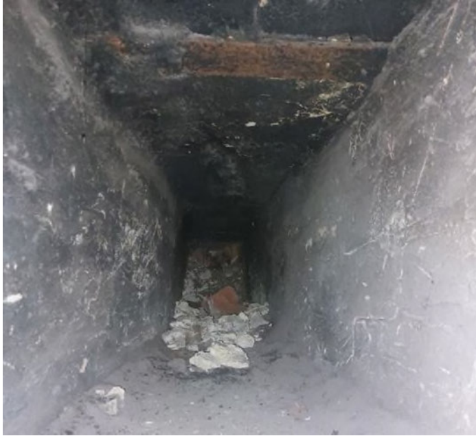
Figure 45 The flue running over the top of the oven chamber.
