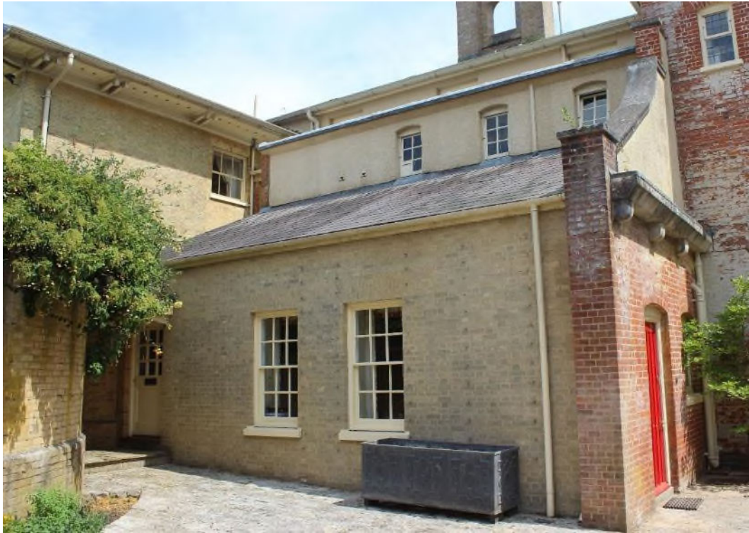
Figure 20 Modern mono-pitched roof addition adjacent to the main part of the Nash house.
