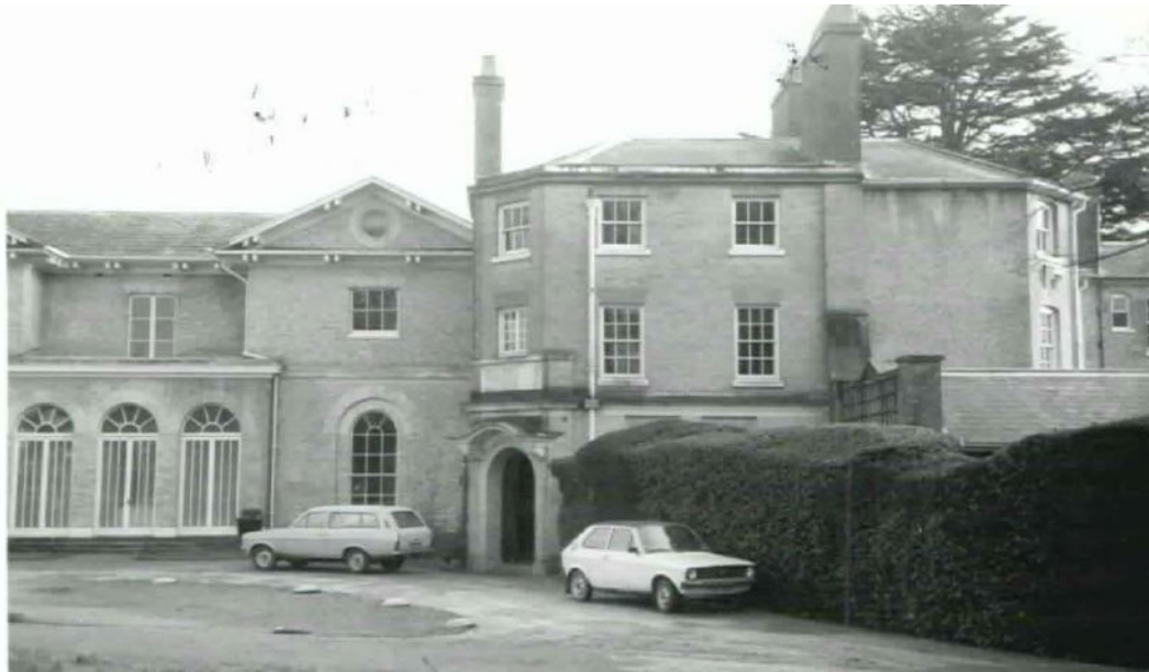
Figure 14 Photo of service block projecting forward of the main front of the Nash House taken before its demolition in 1980. The principal entrance of the house was relocated within this addition.
