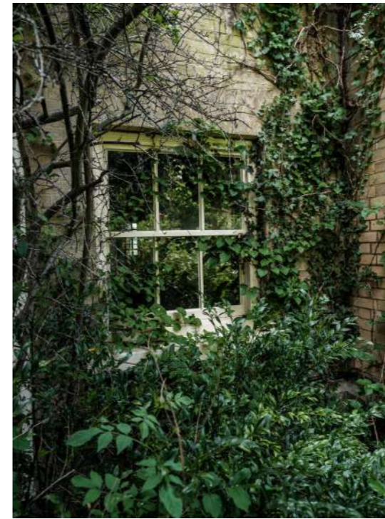
External view of current window
