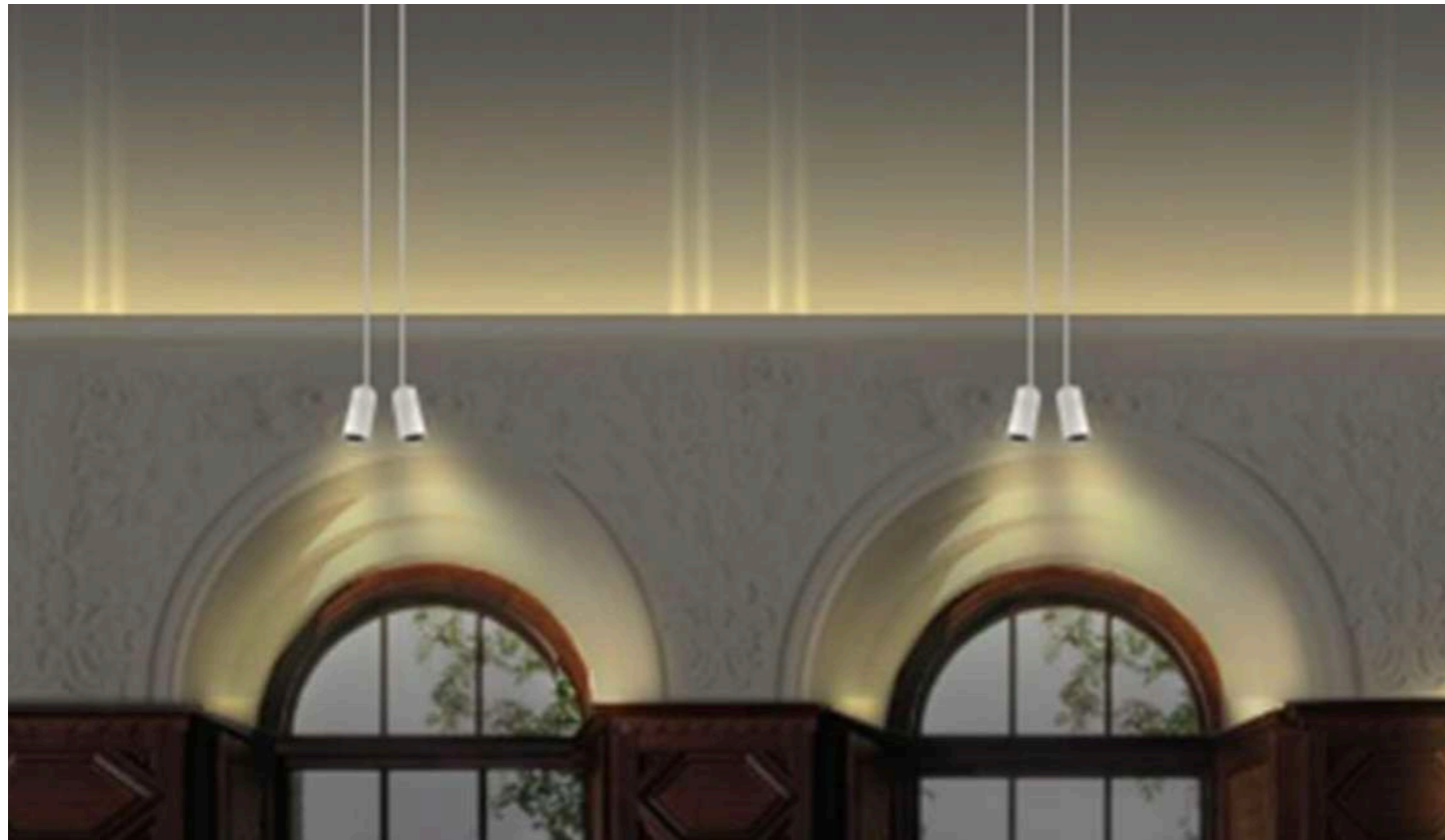
Image of uplit vaulted ceiling with small spot lights to arches and suspended spot lights
