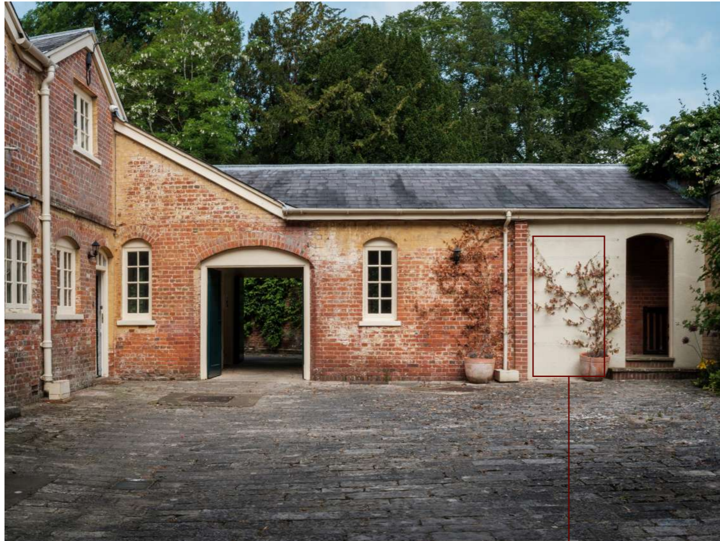
Photograph of service courtyard elevation
