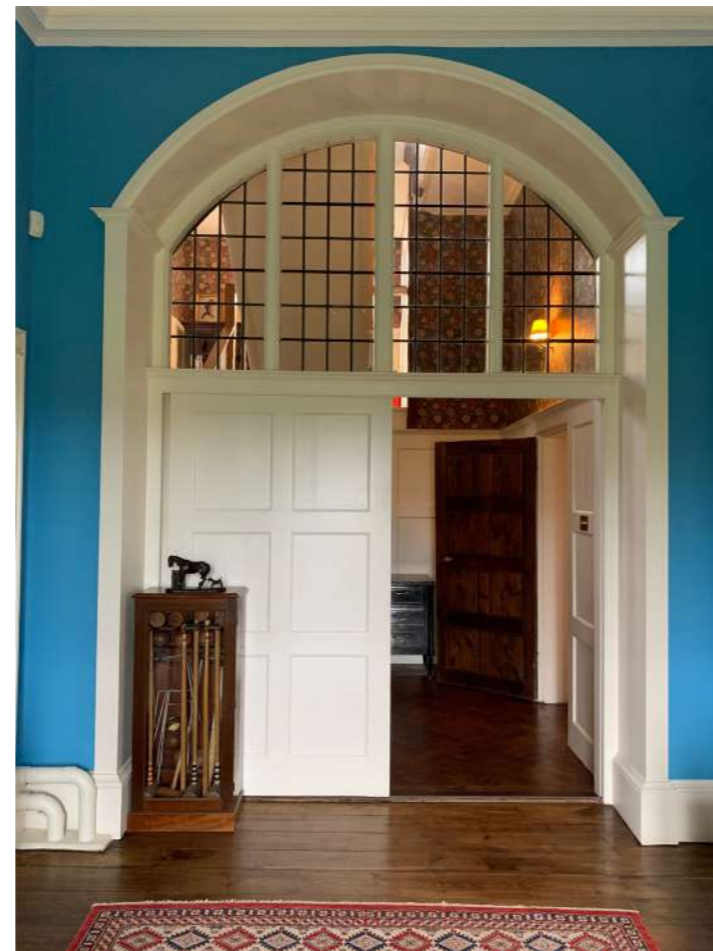
Adjacent sliding screen facing the garden lobby.
