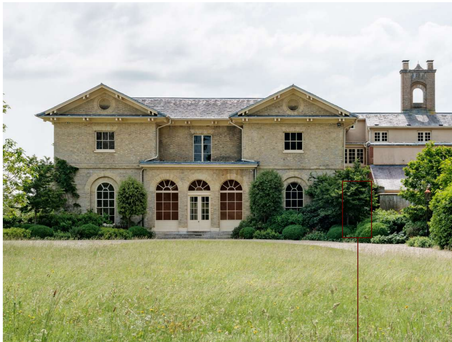
North West Facade
