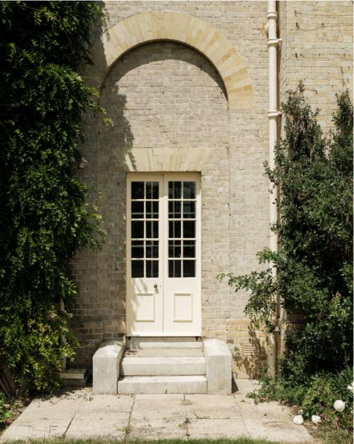
2. Detail of steps on South East Elevation
