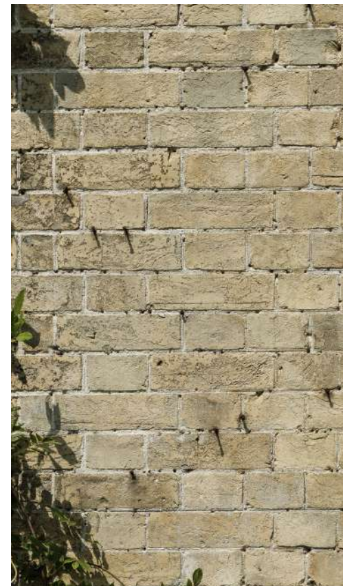
Detail of the original 'Buff' bricks to the Nash House
