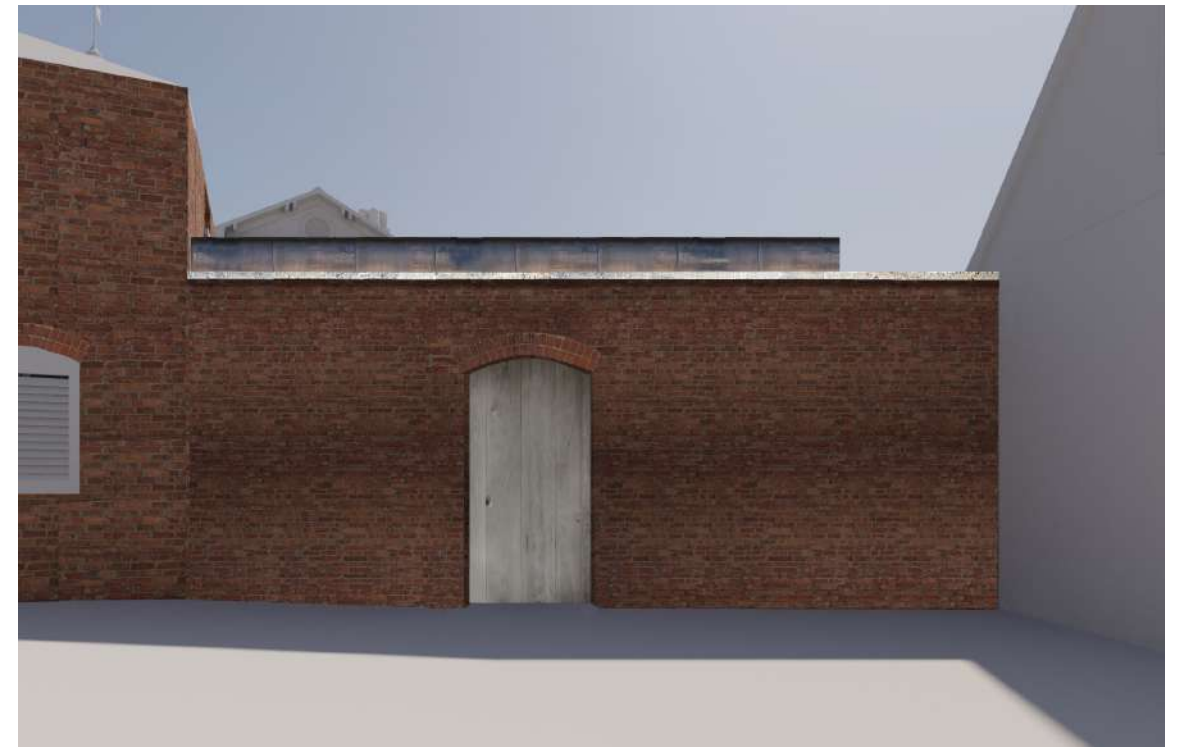
External visual - Existing wall untouched with honed slate panels / set back
