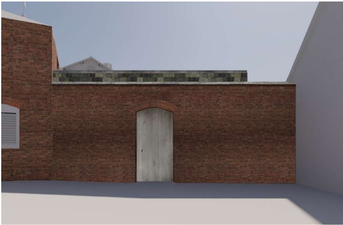
External visual - Existing wall raised with curved coping
