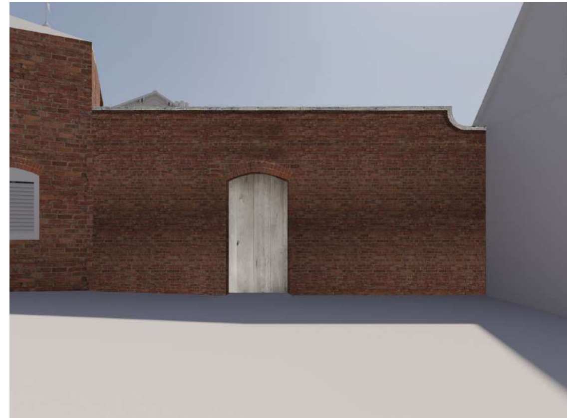
External visual - Existing wall raised with curved coping
