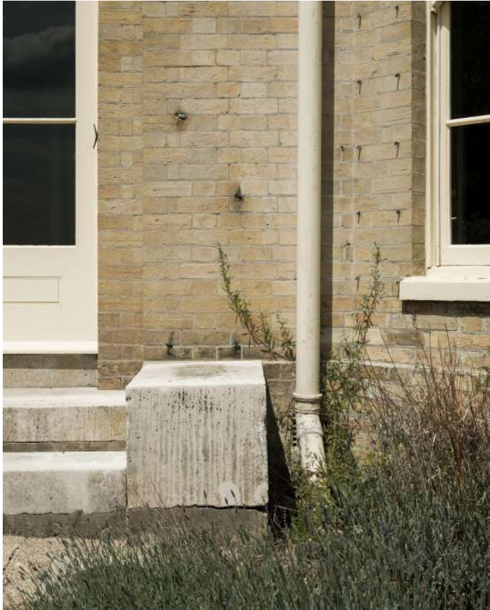
1. Detail of steps on South East Elevation
