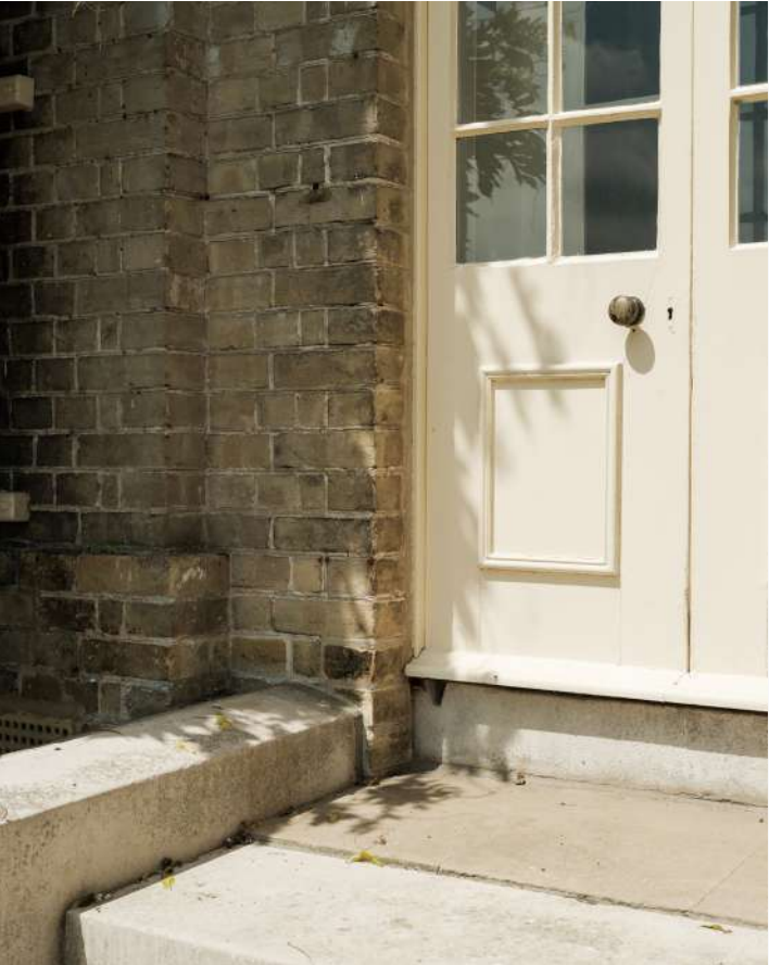
3. Detail of steps on South East Elevation
