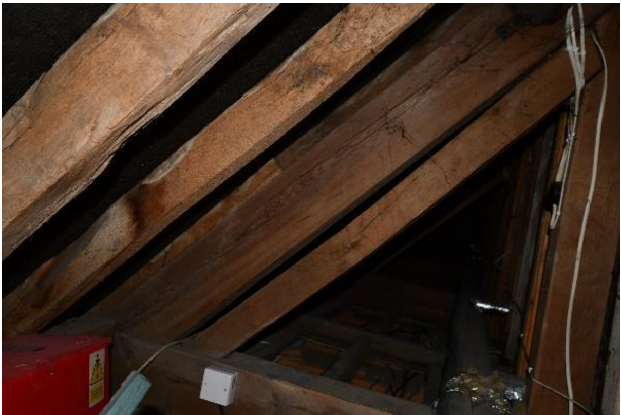
Image 8 Small roof void in Estate Office
