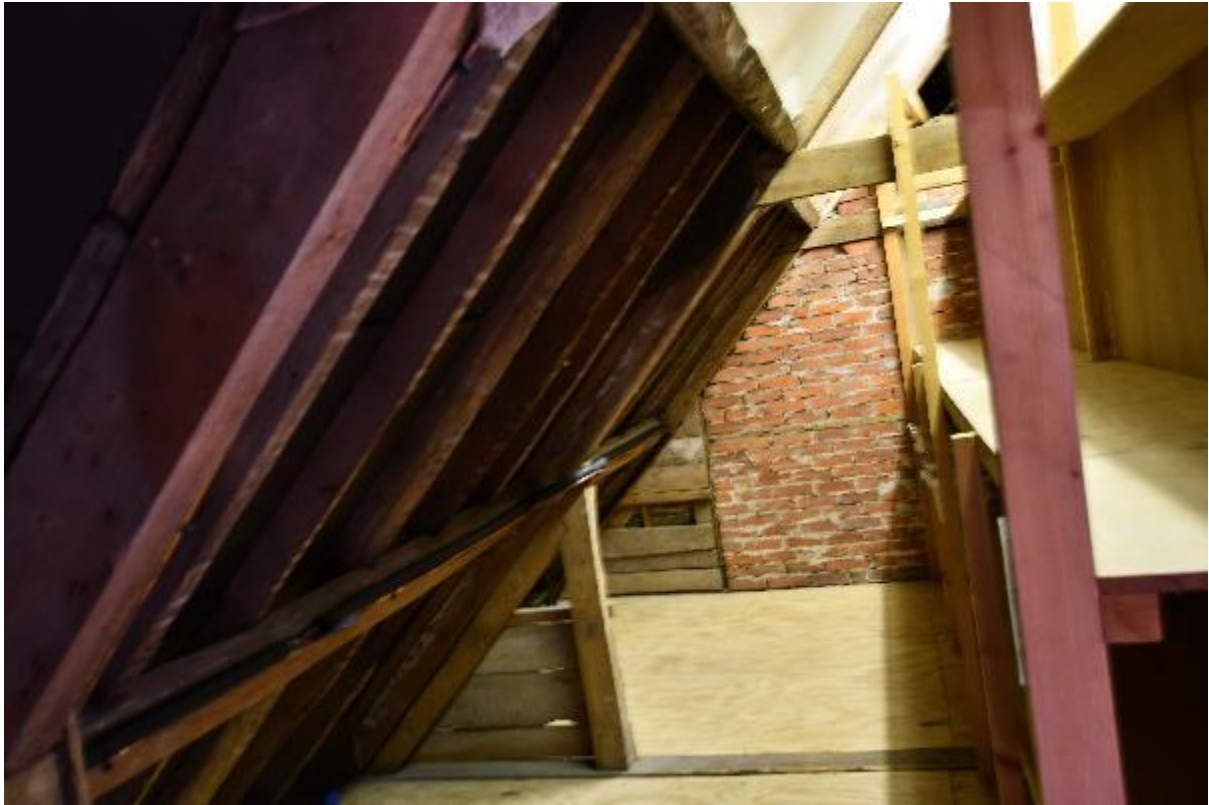
Image 7 Internal structures within Estate Office
