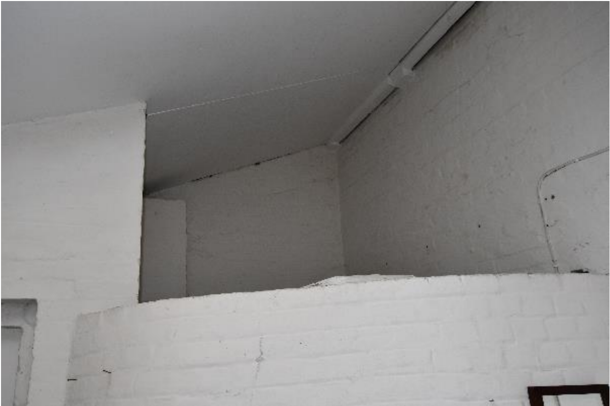
Image 3 Roof structure of Bread Oven
