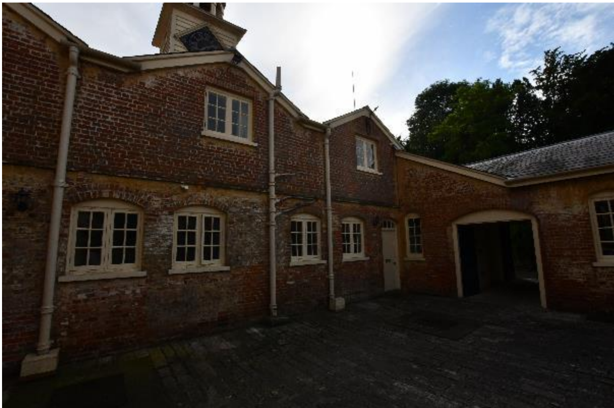
Image 2 Other buildings within courtyard
