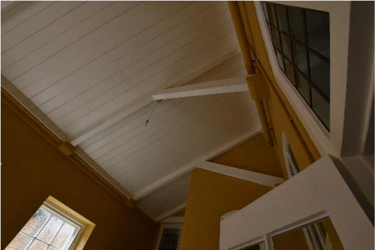
Image 5 Roof structure of Boot Room
