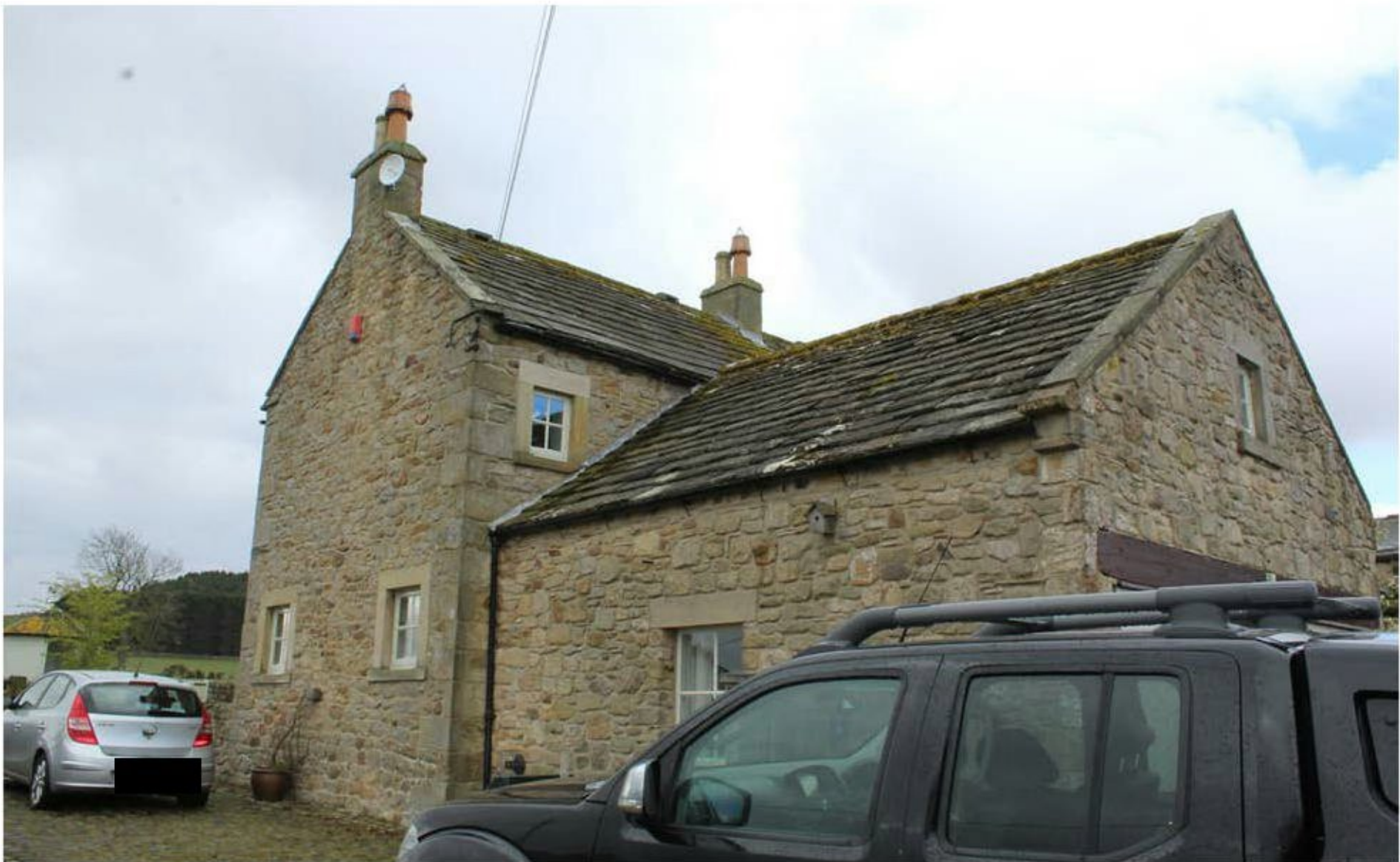
Figure 4 View of garage extension to right, with original farmhouse range to left, looking south-west
