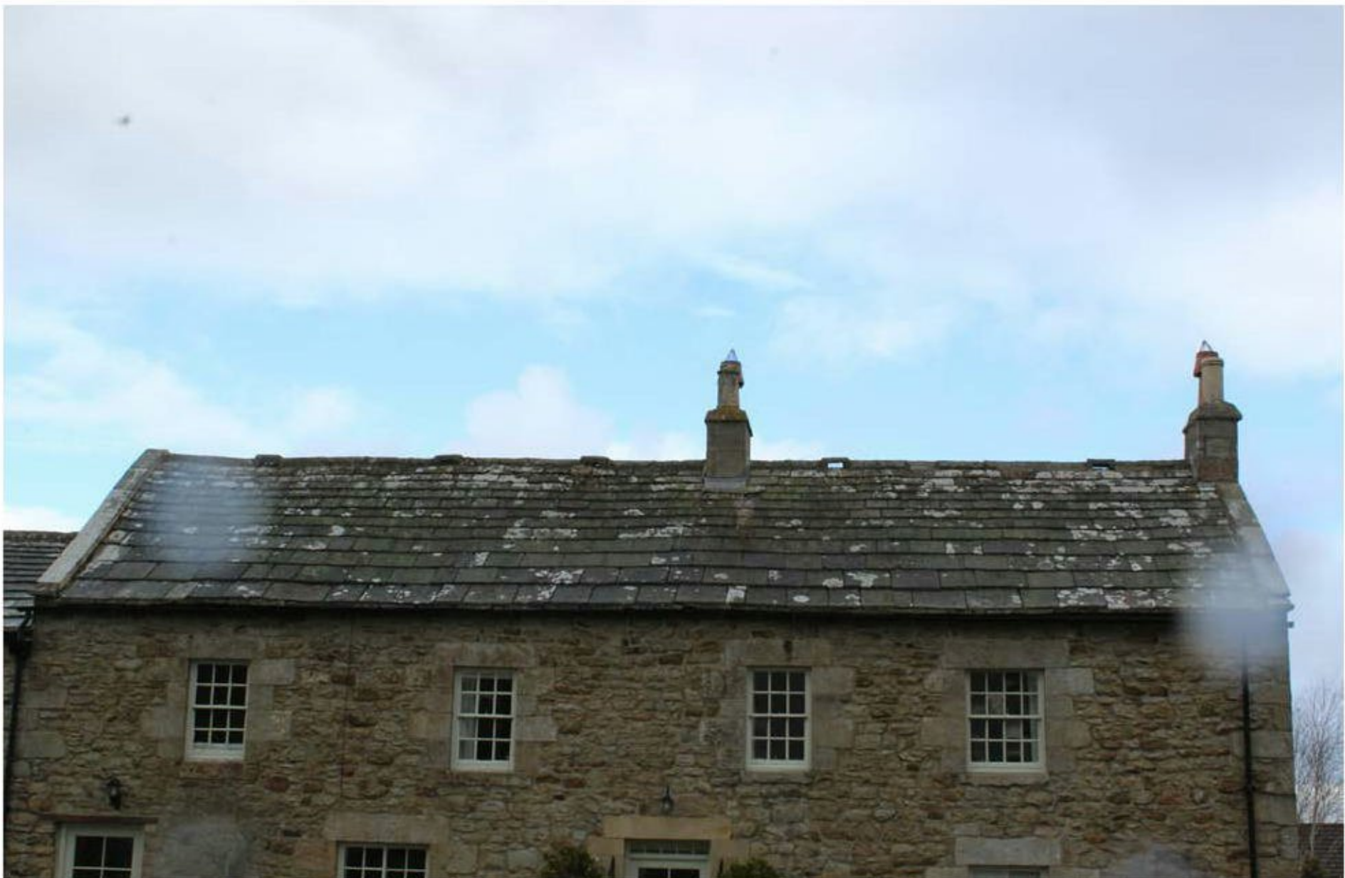
Figure 15 View of ridge of farmhouse range, looking north. Note central rendered chimney stack and ridge vents
