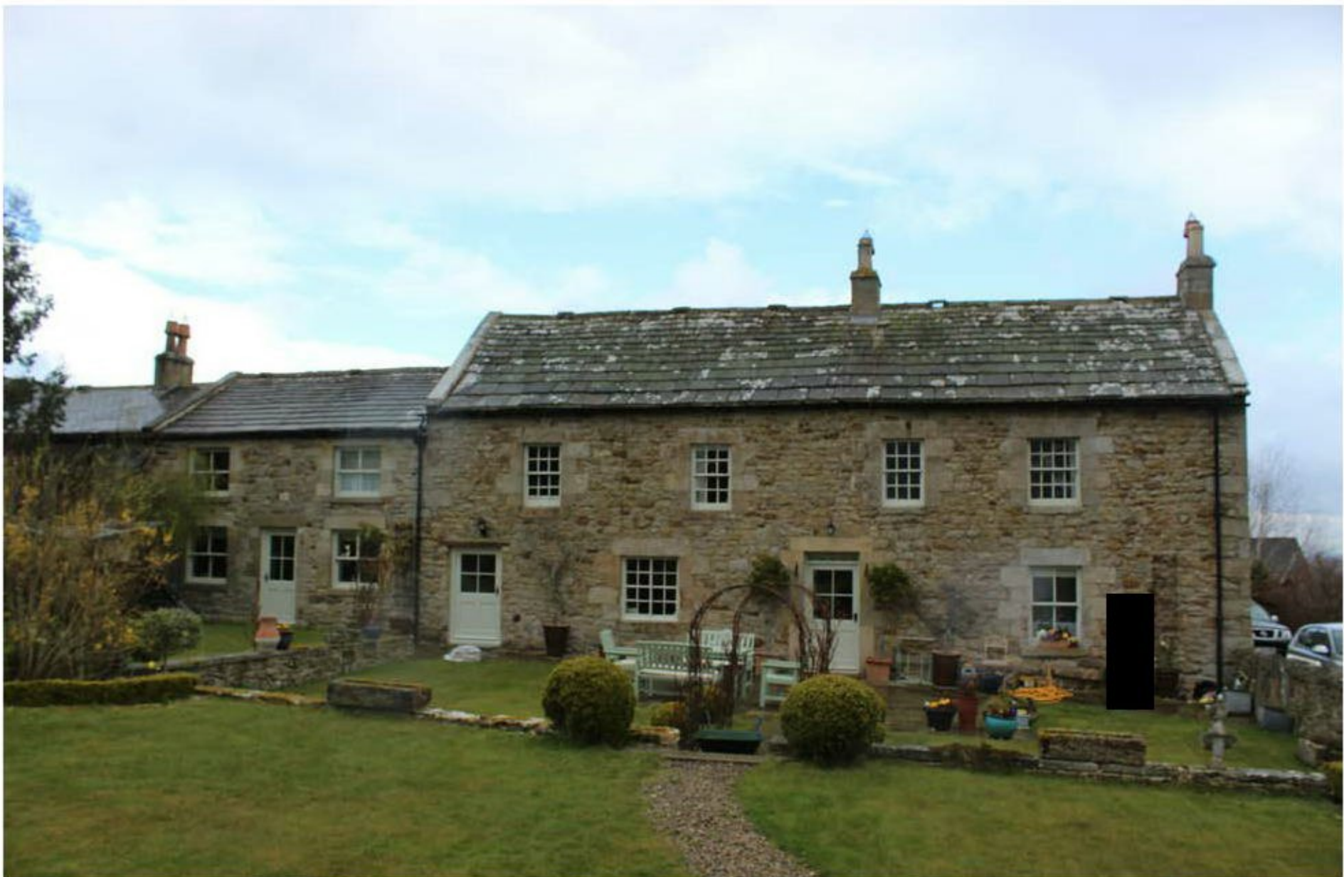
Figure 2 View of principal facade, facing north-west
