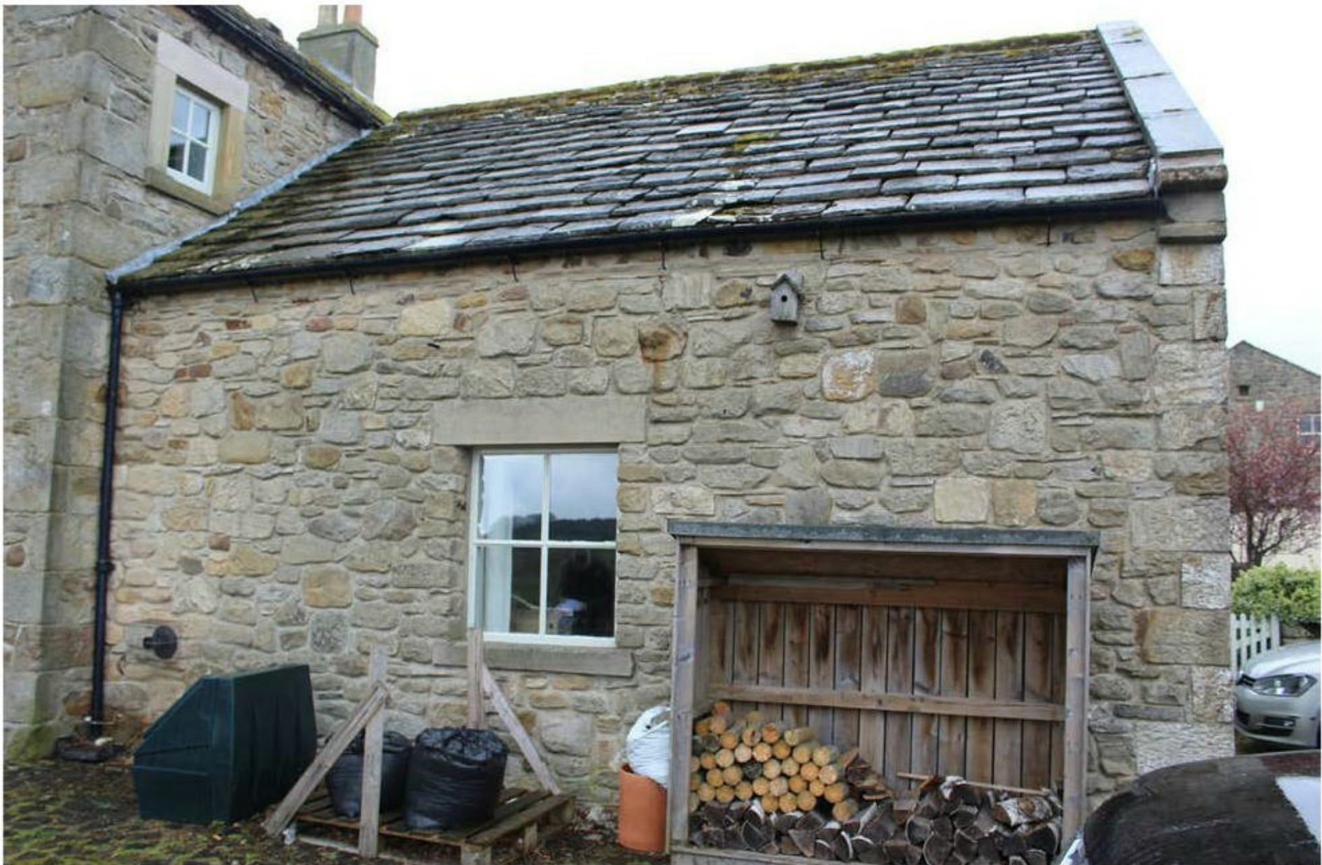
Figure 11 View of window in east elevation of garage extension
