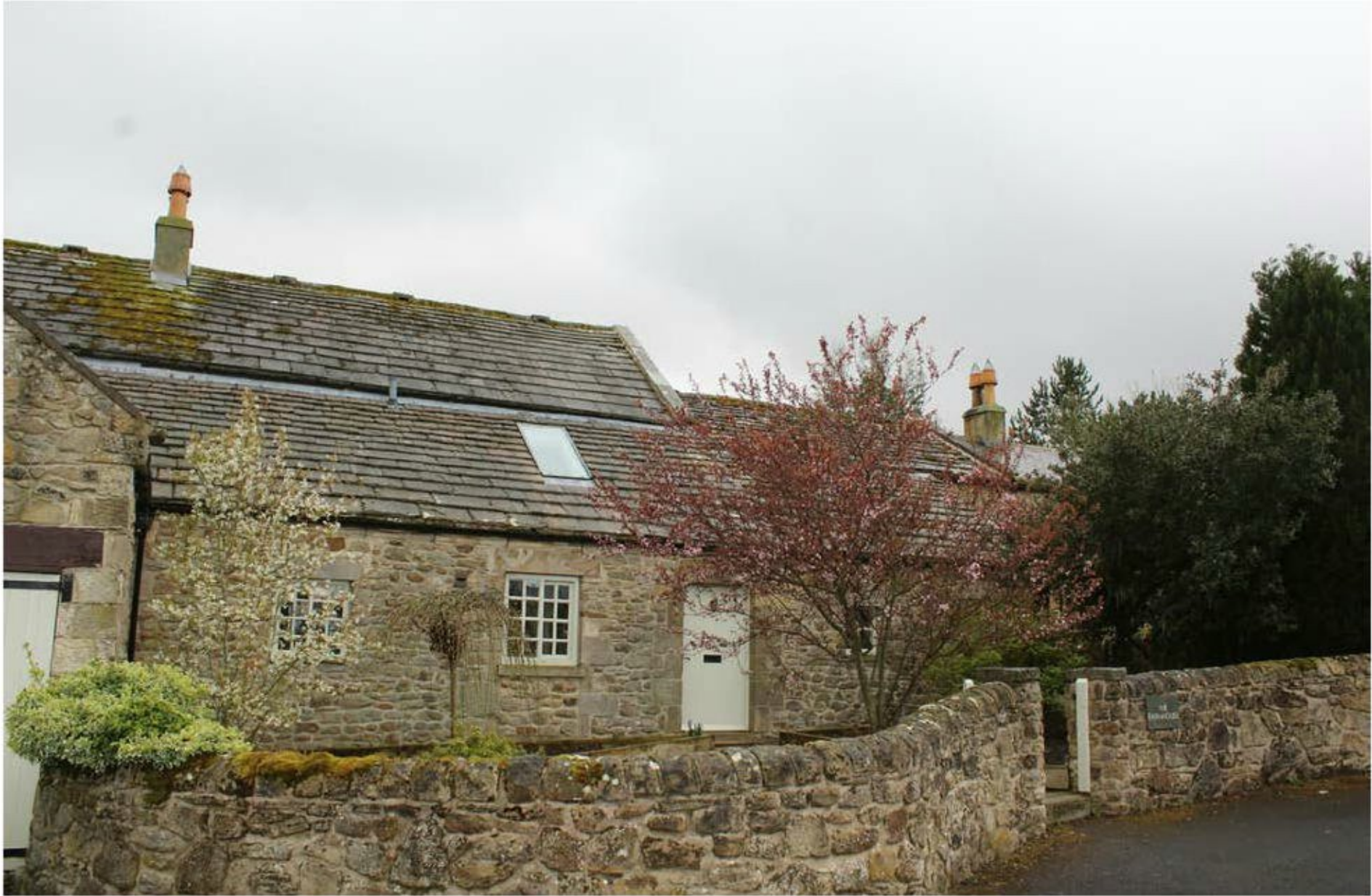
Figure 10 View of rooflight in rear lean-to at north side of farmhouse range
