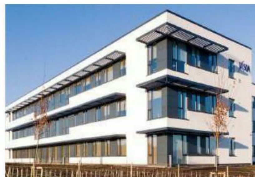
Figure 2: SQA Headquarters (Source: Buccleuch Property)
