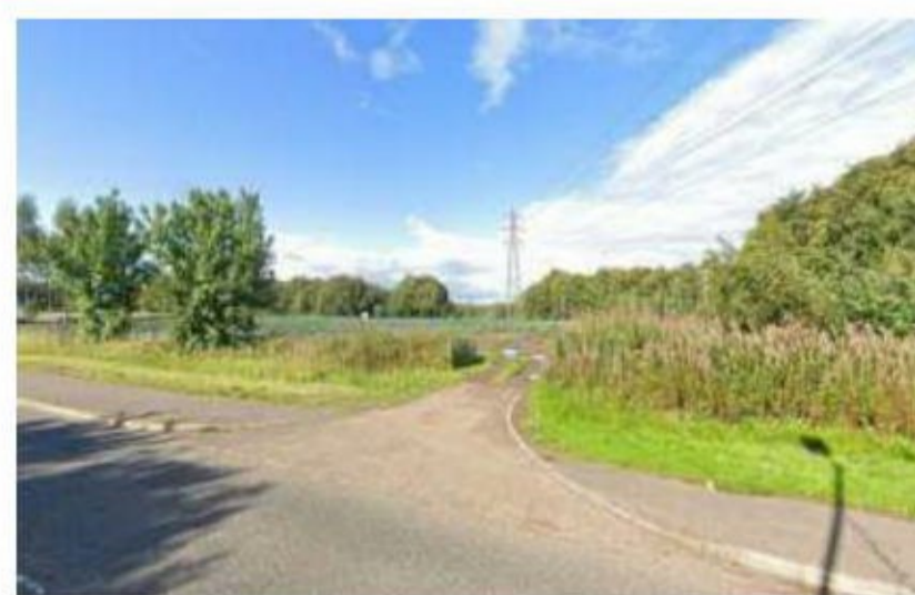
Figure 4: Existing entrance to site from B6392 showing existing overhead cables (Source-Google Maps)
