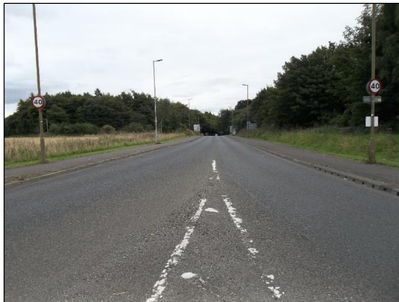
The B6392 Gilmerton Road looking eastwards from the A7 Gilmerton roundabout with the application site to the left
