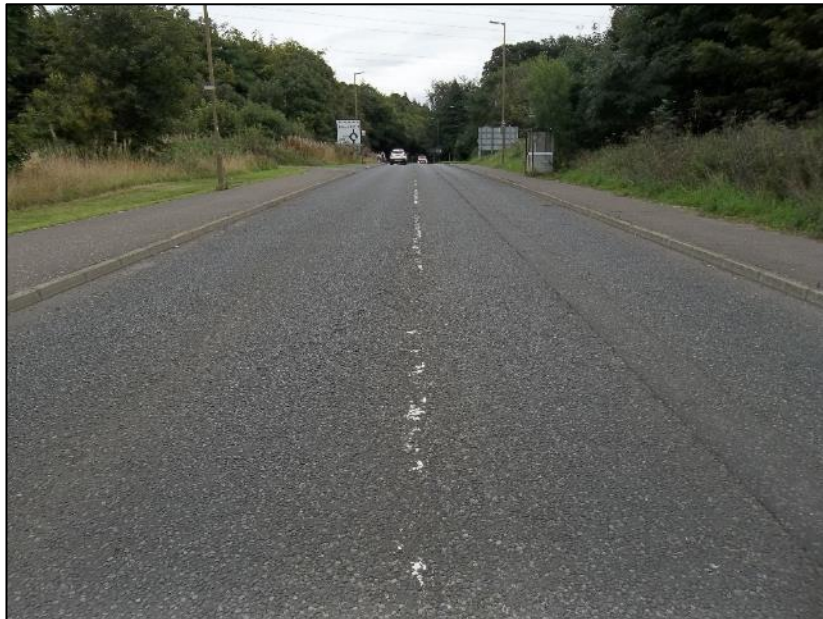
The B6392 Gilmerton Road looking eastwards with the application site to the left
