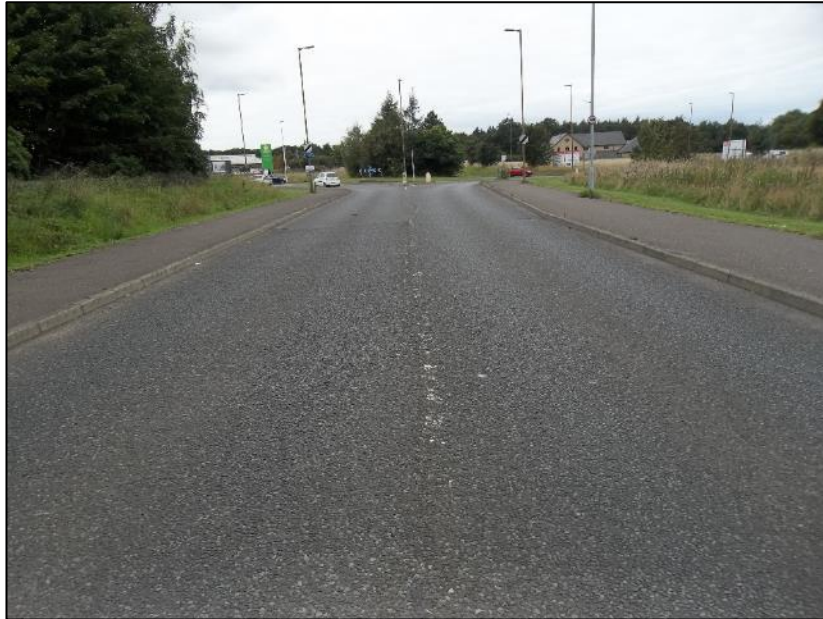
The B6392 Gilmerton Road looking westwards towards the A7 Gilmerton roundabout with the application site to the right
