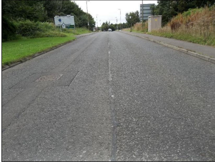
The B6392 Gilmerton Road looking westwards from the Melville Gate roundabout
