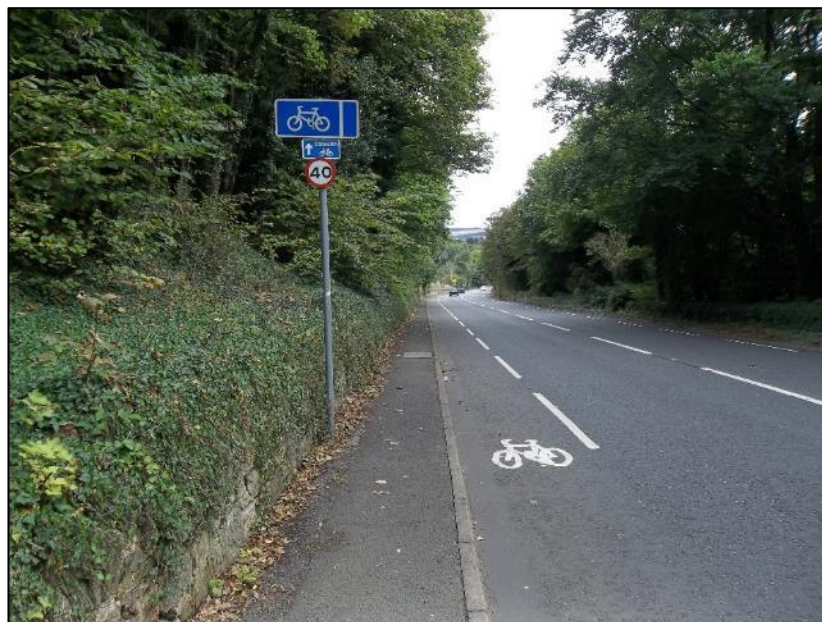
Example of cycle signage and on road provision on the B6392 Gilmerton Road to the south of the Melville Gate roundabout
