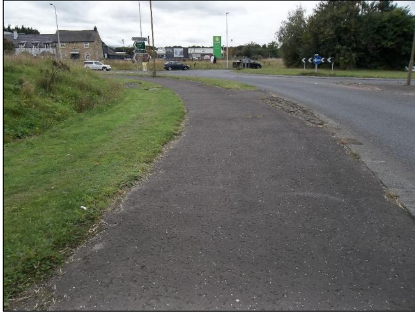
Footway provision along the southern side of the B6392 Gilmerton Road looking westwards towards the A7 Gilmerton Road roundabout
