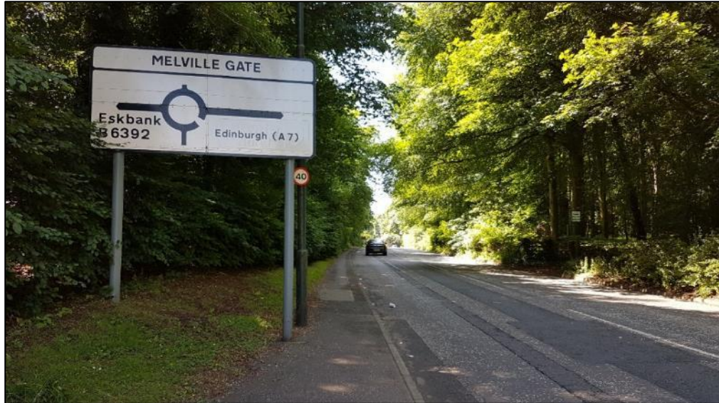
Footway on eastern side of Melville Gate Road.
