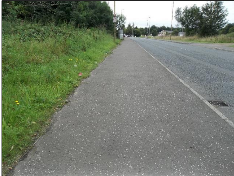
Footway provision along the southern side of the B6392 Gilmerton Road looking westwards with the application to the right
