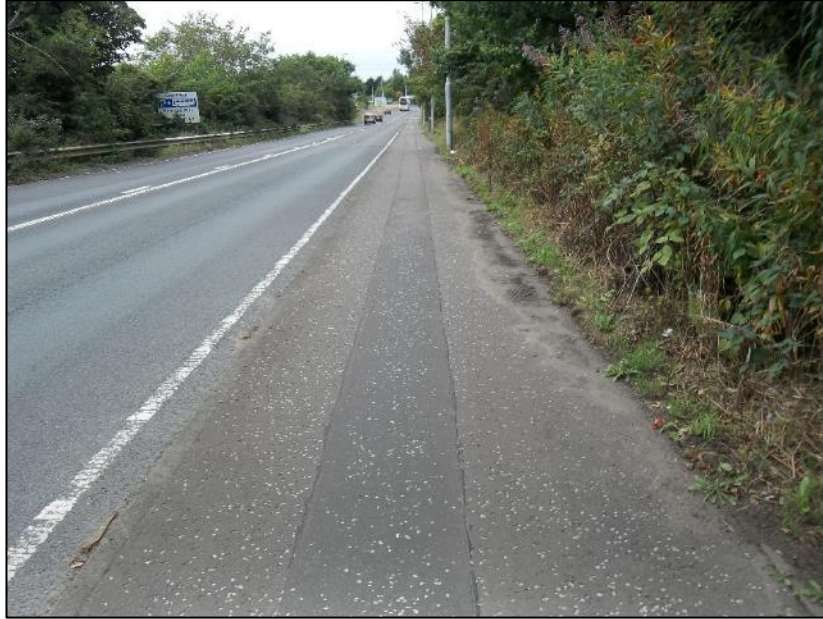
Footway provision along the eastern side of Old Dalkeith Road looking northwards towards Sheriffhall roundabout at the southbound bus stop
