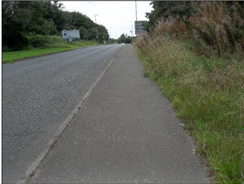
Footway provision along the northern side of the B6392 Gilmerton Road looking eastwards towards the Melville Gate roundabout
