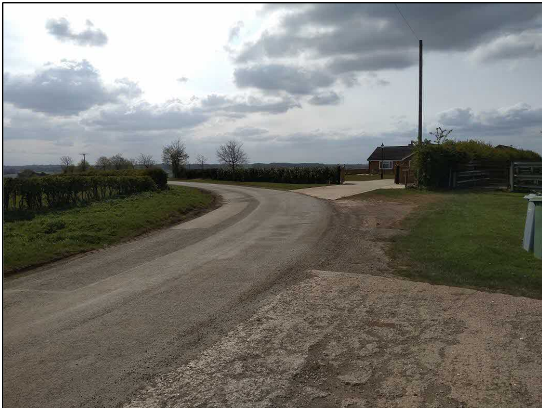
↑ 2) View Southwest along Main Street (from existing access) Note verge overrun owing to absence of entry radii
