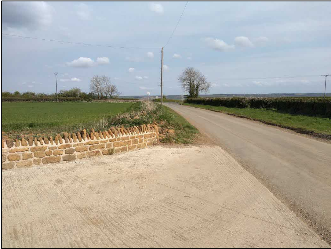
↑ 1) View East along Main Street (from existing access) Note widened access radii and A6003 in rear-of-shot
