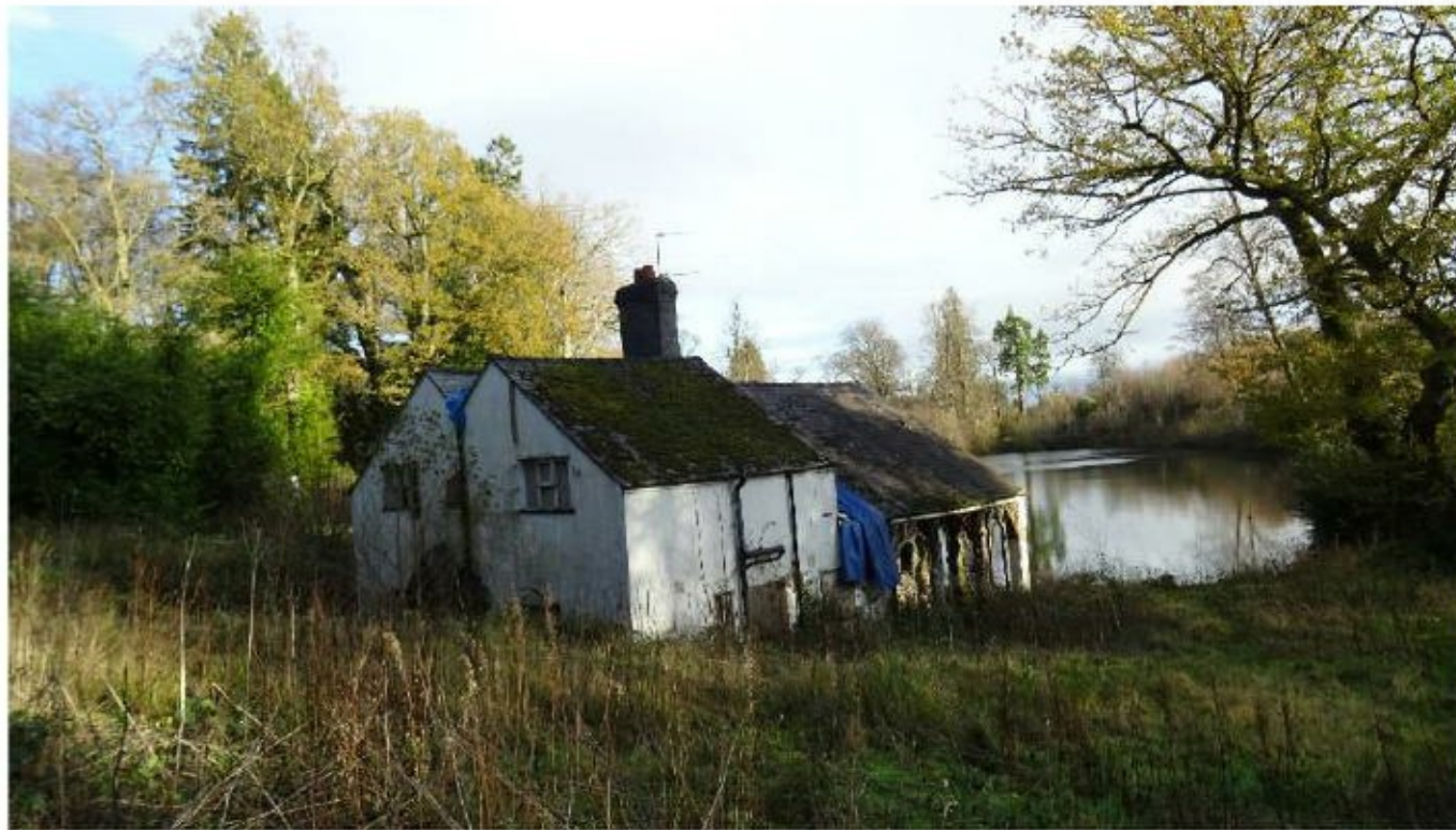
Figure 2.1. Grasses to southwest of building
