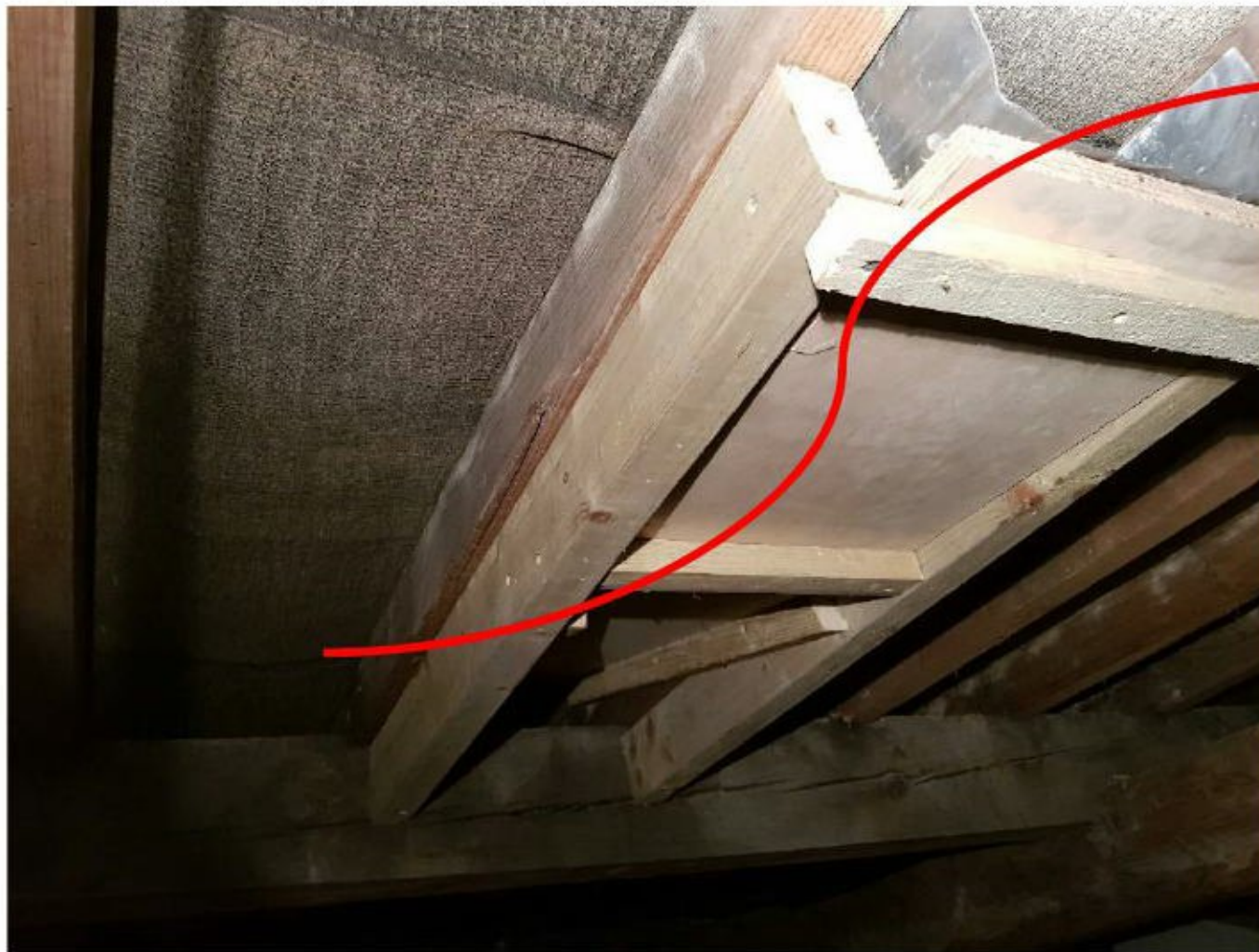
Figure 2.6. Fly-in access internal view (arrow shows proposed flight line)
