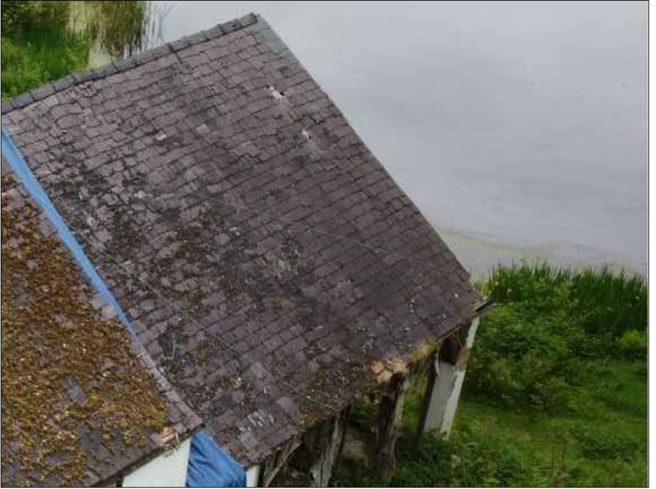
PHOTOGRAPH SHOWING PROPOSED ROOFING MATERIAL: EXISTING ROOF TO BE STRIPPED, SET ASIDE AND RECLAIMED FOR REUSE NEW EXTENSION ROOF TO BE RECLAIMED 20x10 WELSH, HEATHER TONE SLATES TO MATCH MAIN COTTAGE
