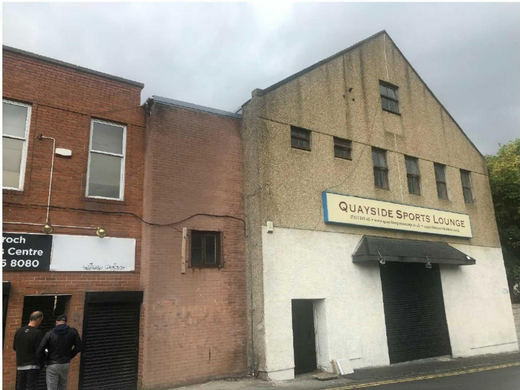
Existing facades to Warroch Street – entrance bottom left of image
