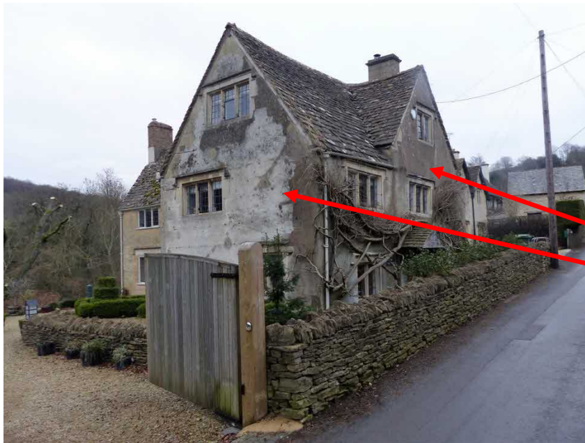
Figure 2 View of the property from the south-west
