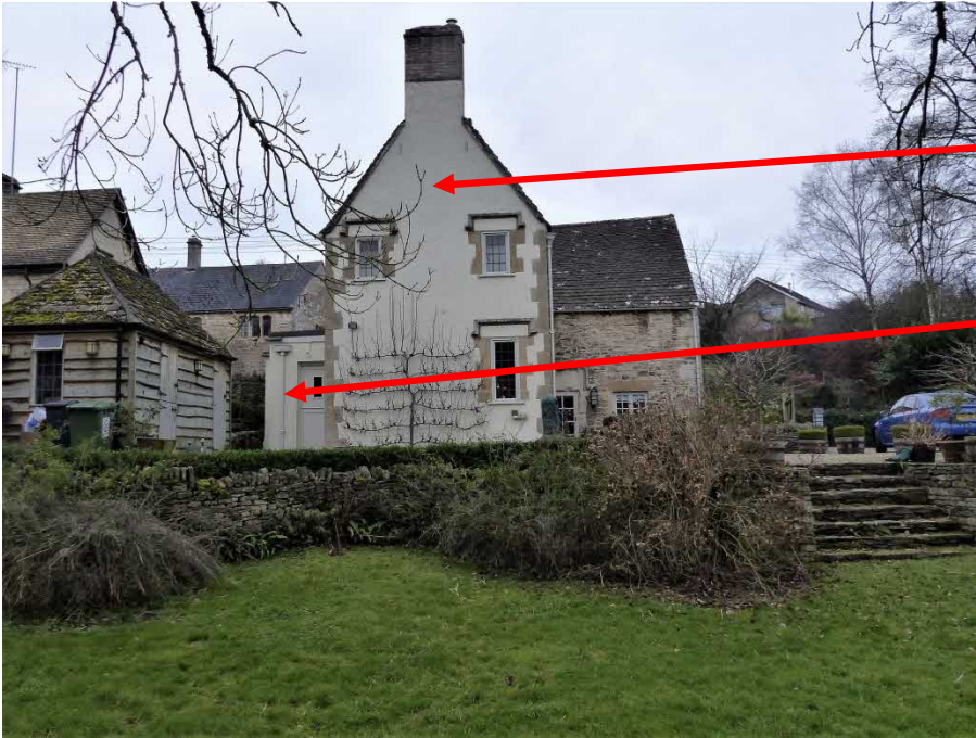
Figure 5 View of the property from the north
