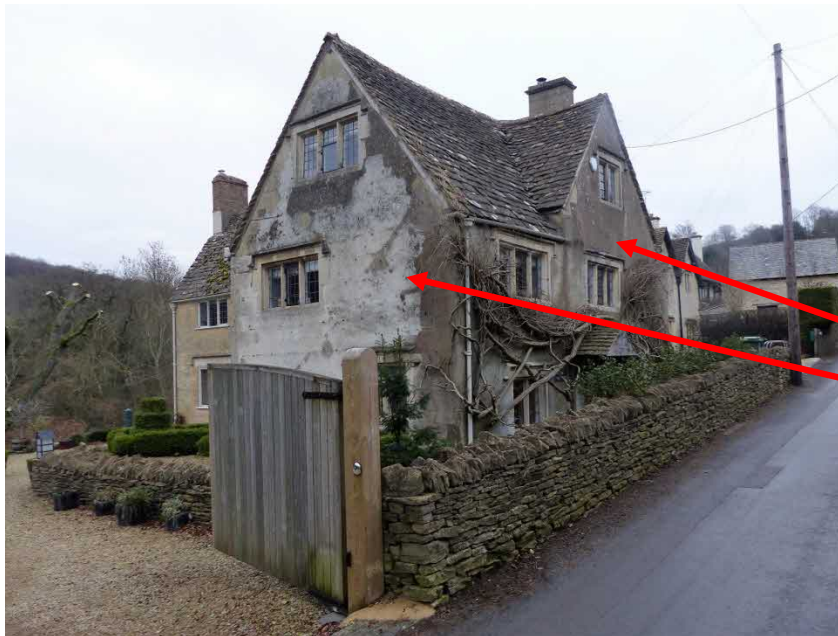
Figure 2 View of the property from the south-west
