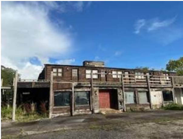
Figure 2.5: Derelict motel in the northern section of the site
