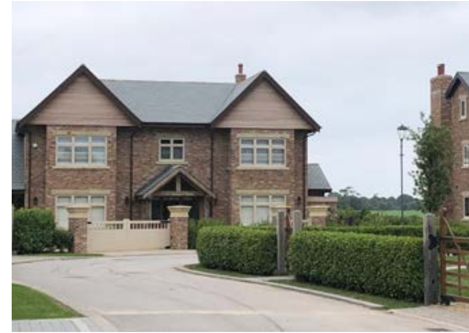
7 - Ballam Oaks, Ballam Road
