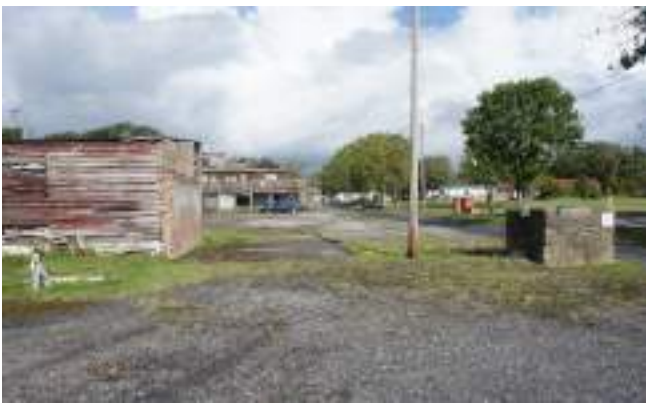
3 Hardstanding and former outdoor dining area
