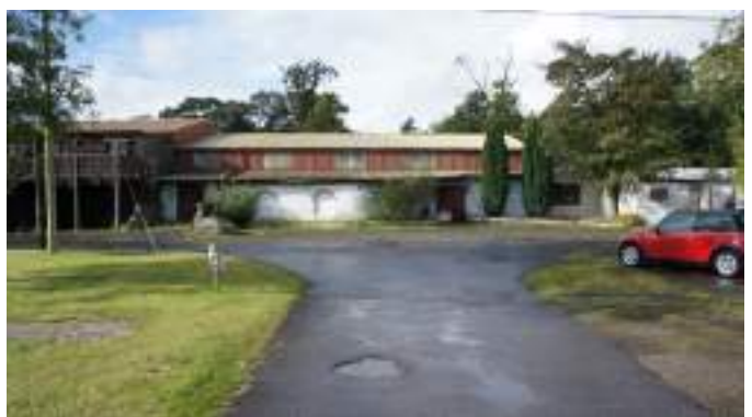
8 View of the eastern elevation of 'Fort San Antone'
