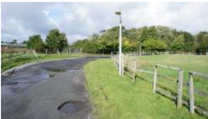
Neglected site infrastructure
