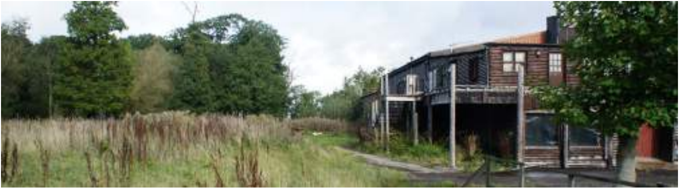
10 View of the western elevation of 'Fort San Antone'
