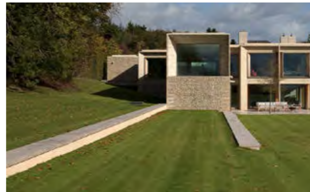
04. Natural stone paving band
