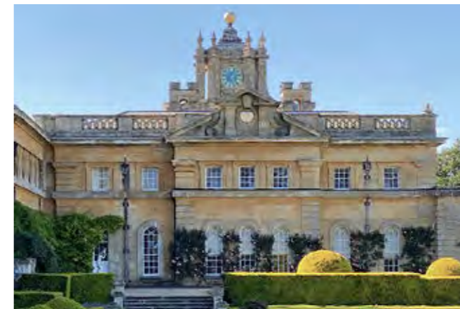
Building and landscape designed as one. Parterre and walled and hedged gardens as outdoor rooms.
