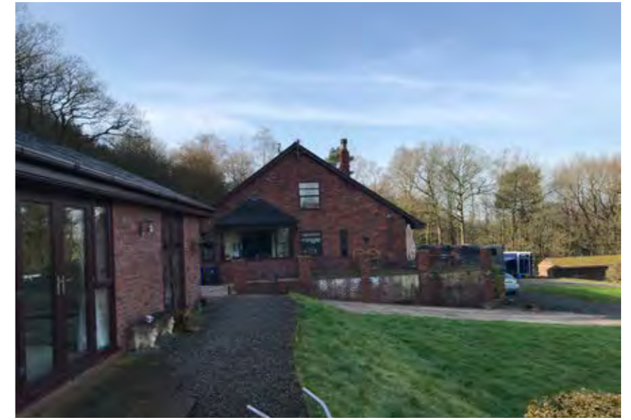
The existing house sits on a substantial brick plinth containing a basement in order to mediate the steep level changes across the site whilst the bungalow sits on plateau created in the falling site. Neither are of architectural significance and both have degraded poorly over time.
