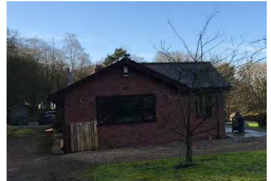
2. The bungalow is of poor architectural quality and badly insulated, offering little to our client.
