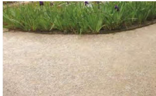
03. Compacted gravel surface
