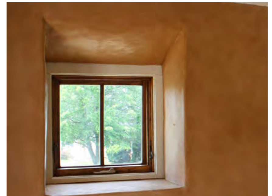
Clay plaster will be used for the inside faces of the external walls, both helping reduce the embodied carbon from cement and facilitating the use of straw insulation, which requires a breathable internal wall finish.
