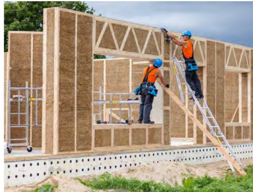
400mm of straw insulation and 60mm of wood fibre board are proposed around the perimeter of the building, necessary to create such a super-insulated building as well as significantly reducing embodied carbon.
