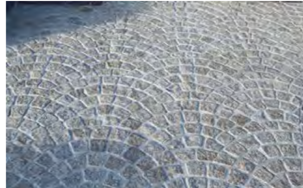
02. Natural stone sett paving
