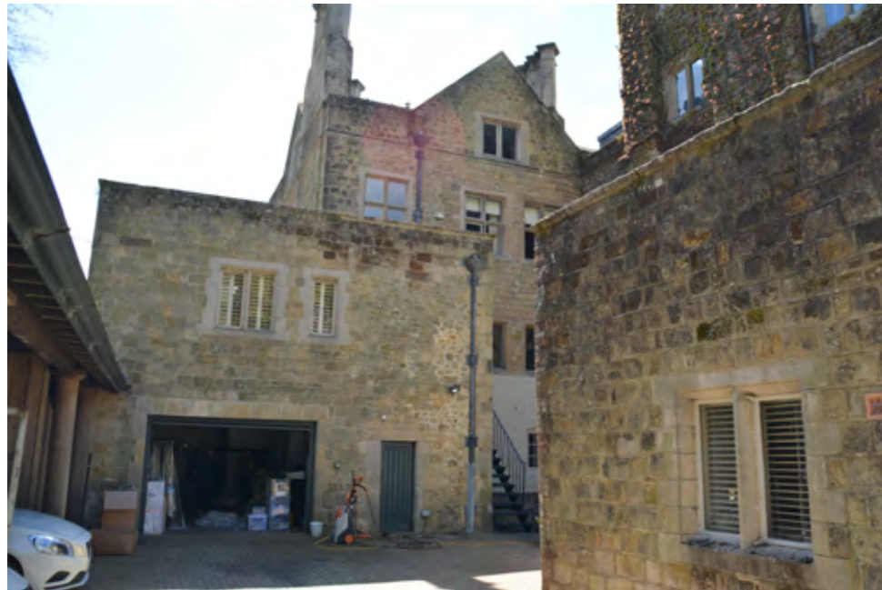
6: General view of the service yard.
