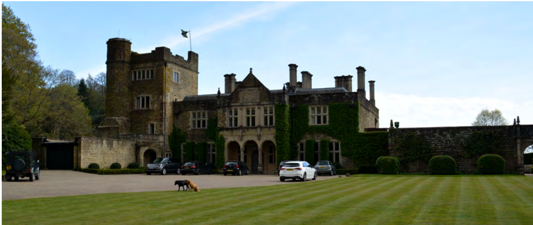
The north elevation of Hollycombe House today. The various demolitions are discussed overleaf.
