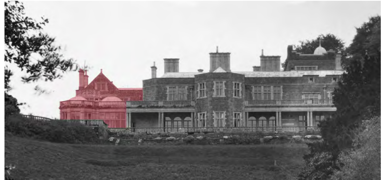
Photograph dated 1932 of the south elevation of the house showing the west wing extension marked up in red. The structure was three storeys to the north with a single storey conservatory to the south lit by a series of glass domes.
