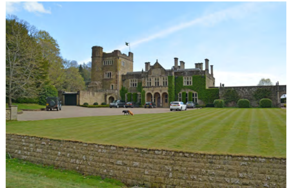
1: General view of the north elevation.
