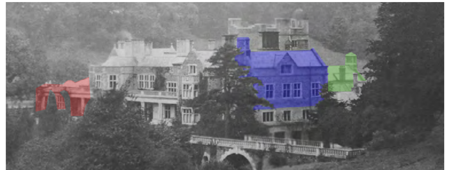
Undated early 20th century photograph from the east showing the west wing (red), east wing (blue) and north wing (green) all demolished by Lord Rea in the mid-1930s.
