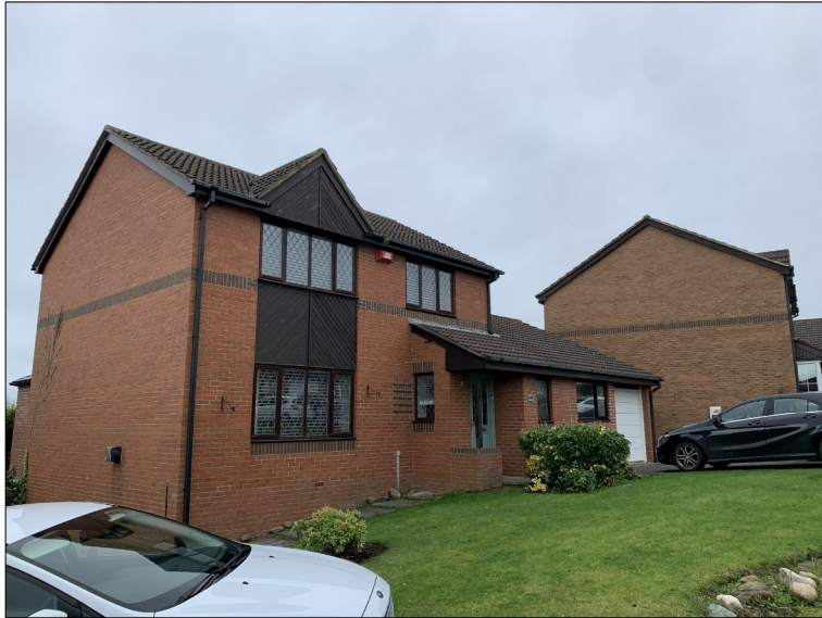
Photo 1 : Front view of 60 Turnberry looking south eastwards
