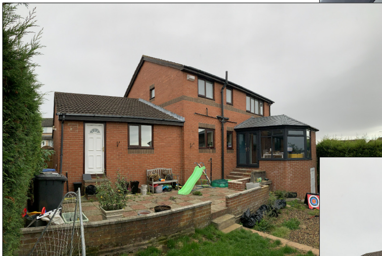
Photo 3 : Rear view looking north westwards
