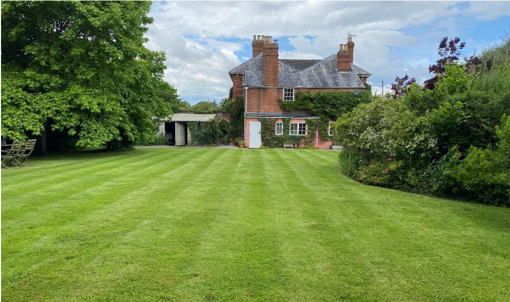
View of the east elevation from the rear garden
