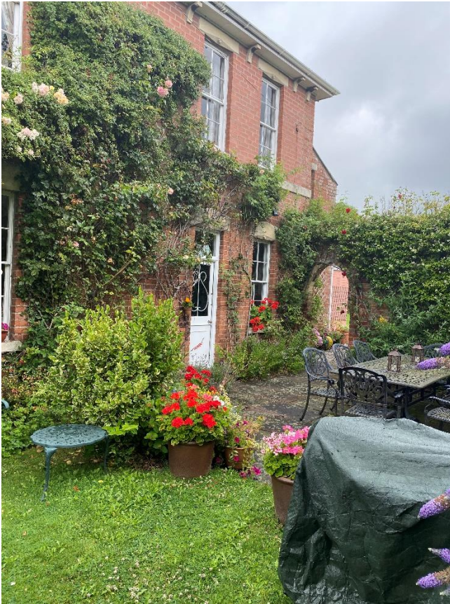
Existing south elevation of the main house showing the arched opening in the garden wall that is to be removed
