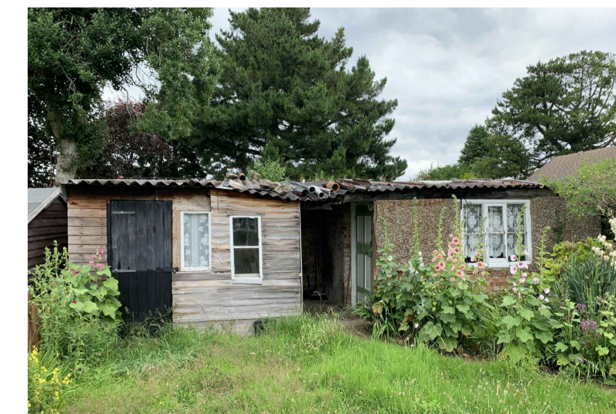
EXISTING GARDEN ROOM (DERELICT) - TO BE REPLACED.
