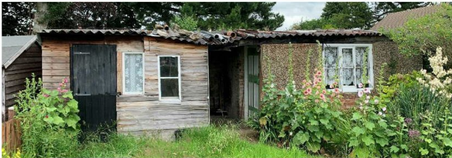
Figure 33 – Existing Garden Room / Potting Shed / Store
