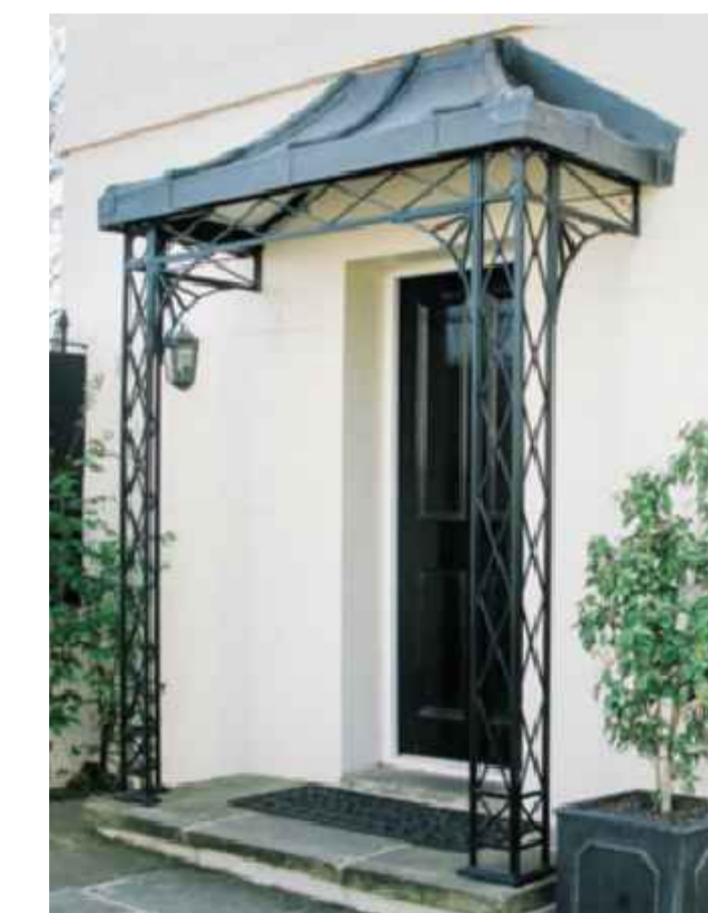
15 - CAST IRON PORCH WITH LEAD ROOF
