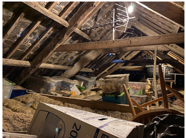
Main Roof Space
