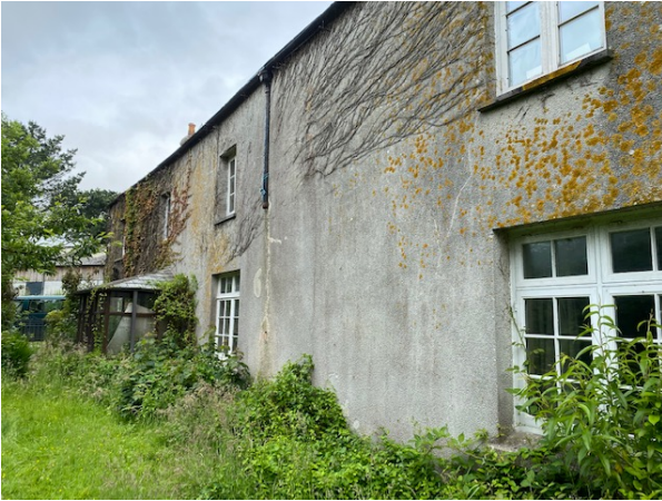
South East Elevation (looking West)
