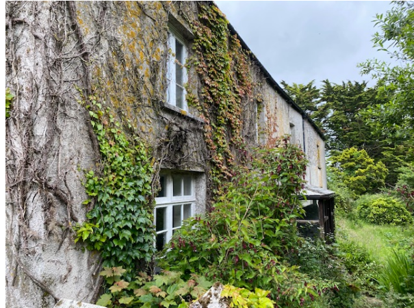
South East Elevation (looking East)
