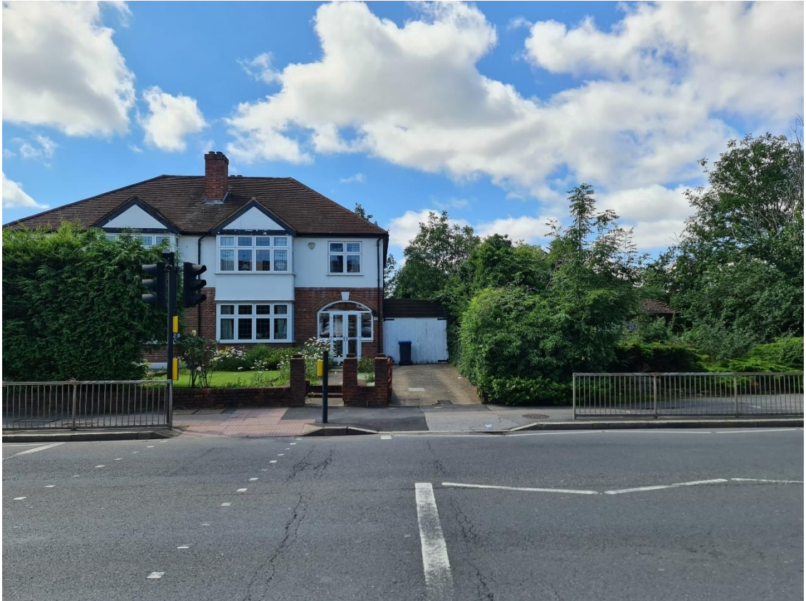
Fig.6: View looking southwest from the north side of Malden Road showing no.375 in context with the development site to the right.
