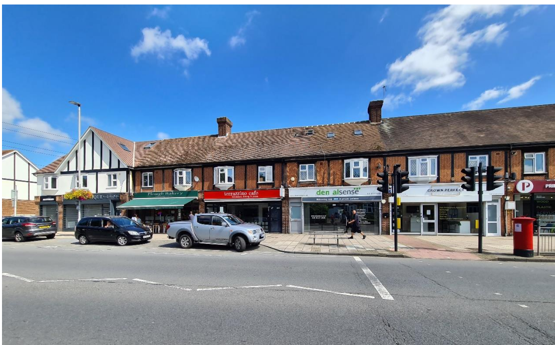
Fig.5: North side of Malden Road, opposite the site's northeast boundary.
