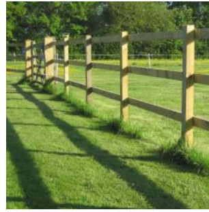
Existing Fence Post and rail fence to be made good
