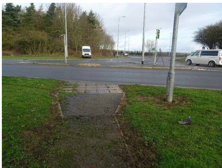
Photo 3: Dropped Kerbs and Tactile Paving at Killingwoldgraves Roundabout
