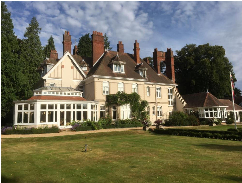
View from garden to the east
