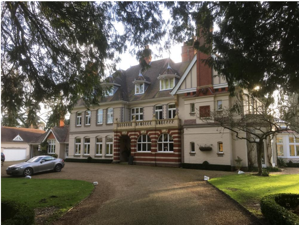
View from entrance drive
