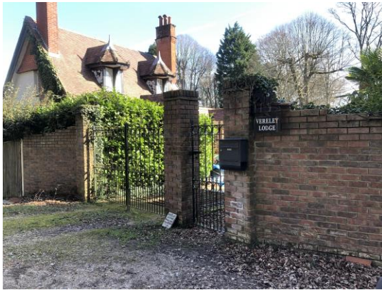
Entrance gates to Vereley Lodge
