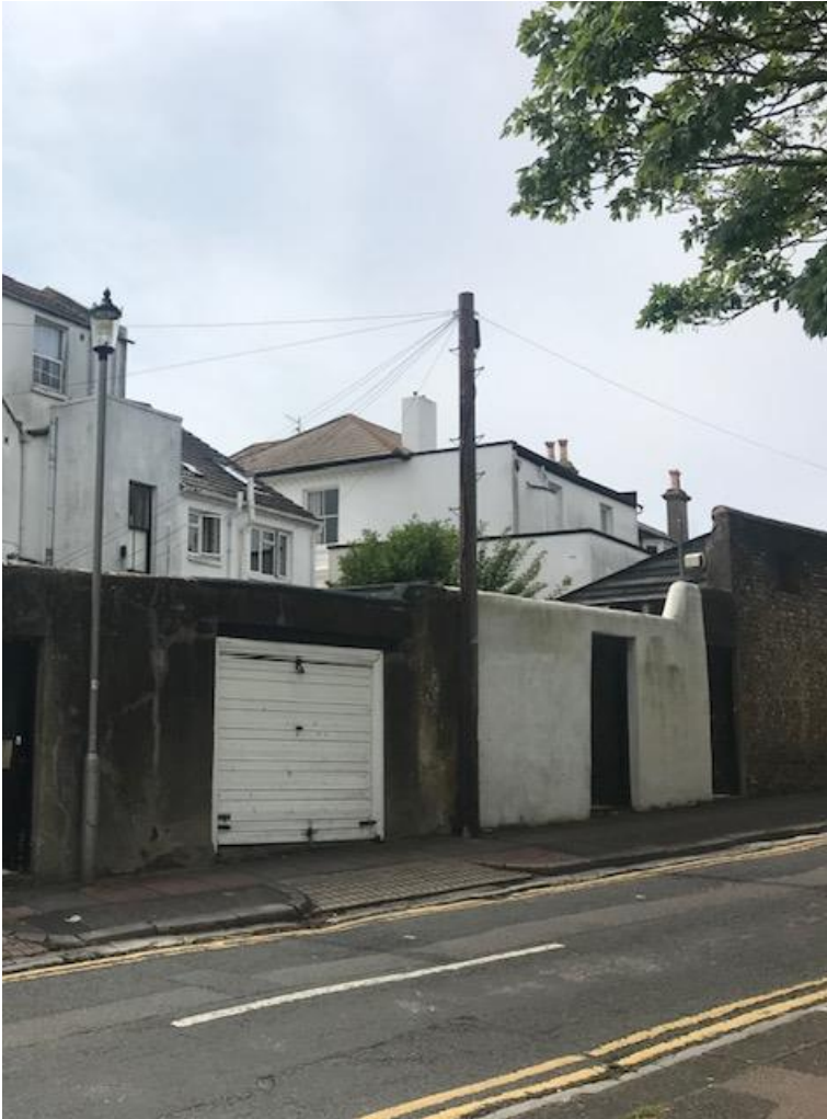
Flat roofed rear additions to both neighbouring dwellings.
