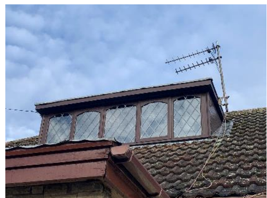
Figure 18. Lifted lead flashing around dormer window and porch roof on the southern elevation of the main house (B1)
