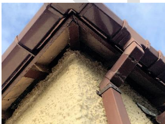
Figure 17. Gap between external wall and eaves on southeast corner of the main house (B1)
